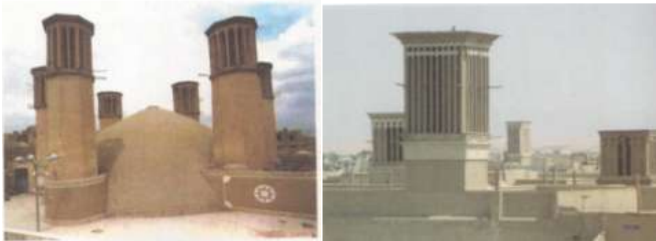
Figure 37: Water reservoir & wind catchers in Yazd city
