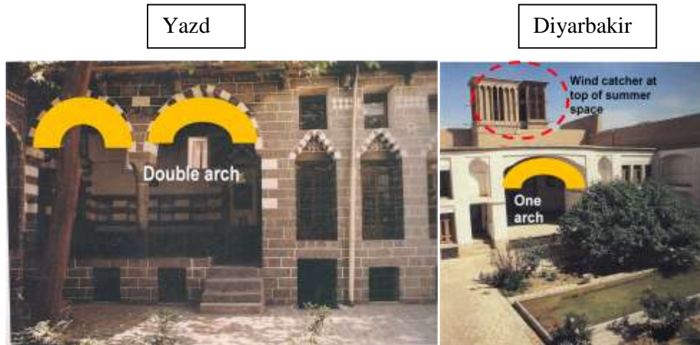
Figure 62: Different forms of semi open spaces in Diyarbakir and Yazd regions (Tuncer,1999)
