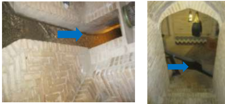
Figure 39: Cellar in Yazd old houses
