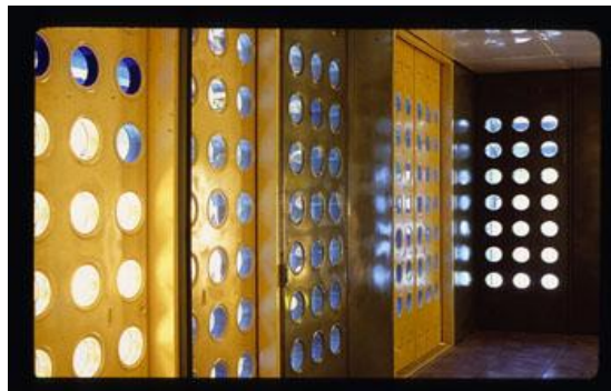
Figure 2: Folded sheet metal in the interior of Prouve's house (Source:www.designmuseum.org)
