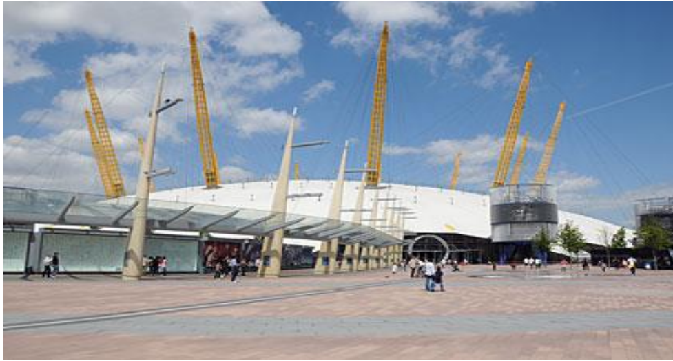
Figure 25: Millennium Dome Entrance (Source: www.wikipedia.com )
