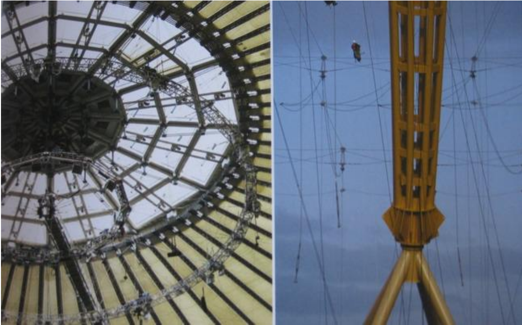
Figure 26: Detail of the structure of the mast (Source: www.arcspace, com )
