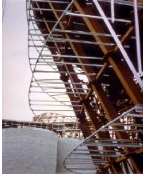
Figure 29: Atrium with primary, three-meter structural grid (Source: www.arch.ethz.ch )
