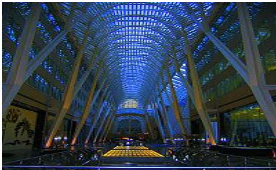
Figure 12: Ribbed Structure shown in Allen Lambert Galleria (Source: http://eng.archinform.net )
