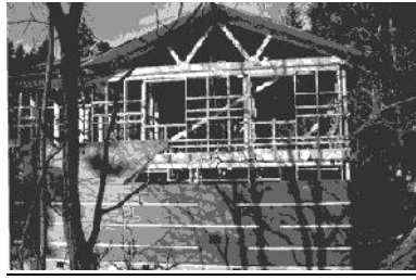
Figure 3.2 Wooden balloon system [Schömer G.E., 1977]
