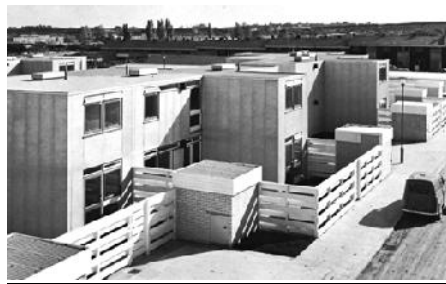
Figure 3.3 Lightweight concrete system [Schömer G.E., 1977]
