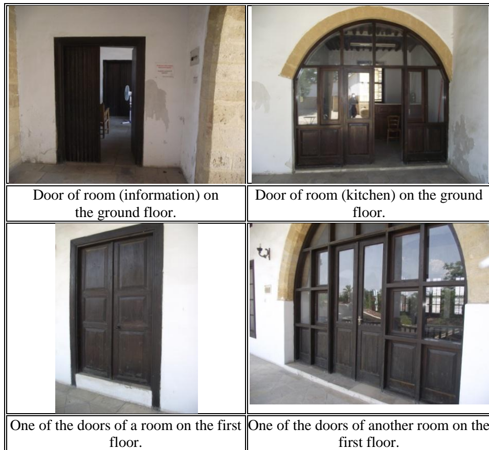
Figure 119: Doors at the semi-open spaces, Lusignan House (Author, 2012).
