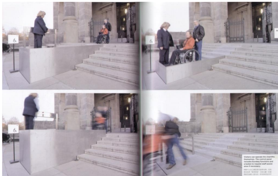
Figure 1: Retractable access lift, Bode Museum, Berlin (Fischer and Meuser, 2009, p: 114-115).
