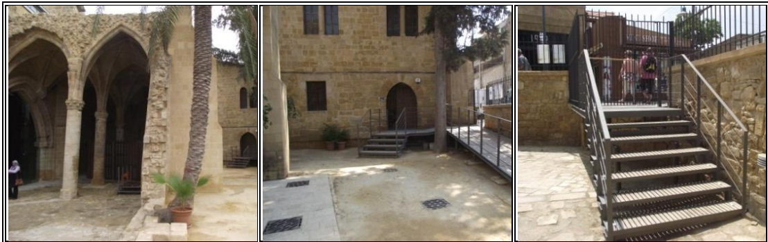
Figure 99: Steps and stairs in the defined open spaces, Bedesten (Author, 2012).
