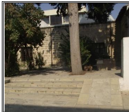
Figure 56: Ramp in the defined open spaces, Mevlevi Tekke Museum (Author, 2012).
