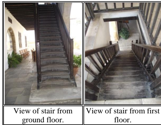
Figure 107: Stair at the semi-open space, The Eaved House (Author, 2012).
