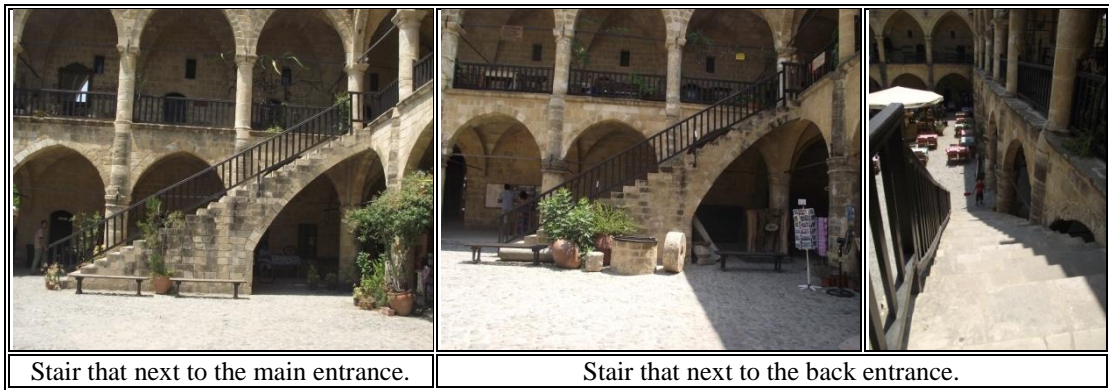
Figure 87: Steps and stairs in the defined open spaces, Great Khan (Author, 2012).
