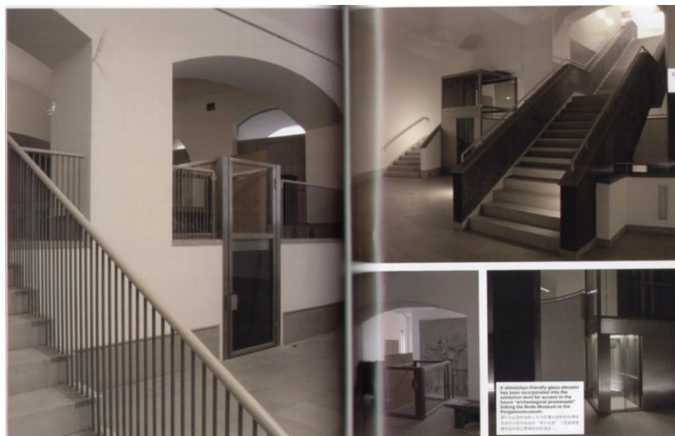
Figure 2: Through floor lifts, Bode Museum, Berlin (Fischer and Meuser, 2009, p: 118-119).
