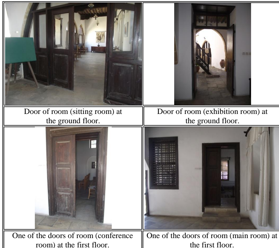
Figure 106: Doors at the semi-open spaces, The Eaved House (Author, 2012).
