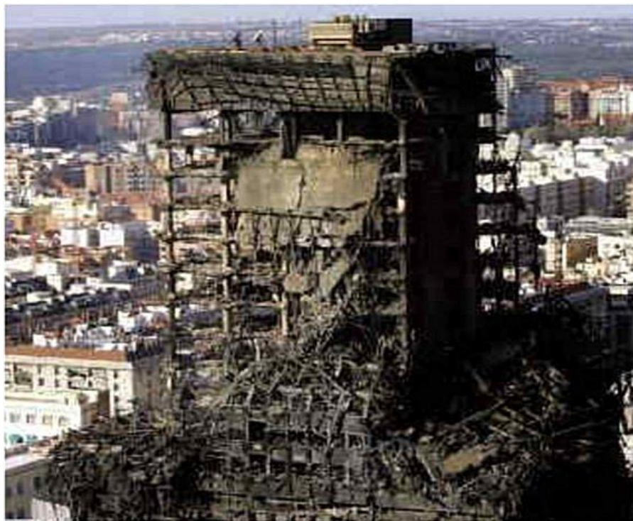
Figure 3. The Windsor Tower, Madrid, Spain [13]
