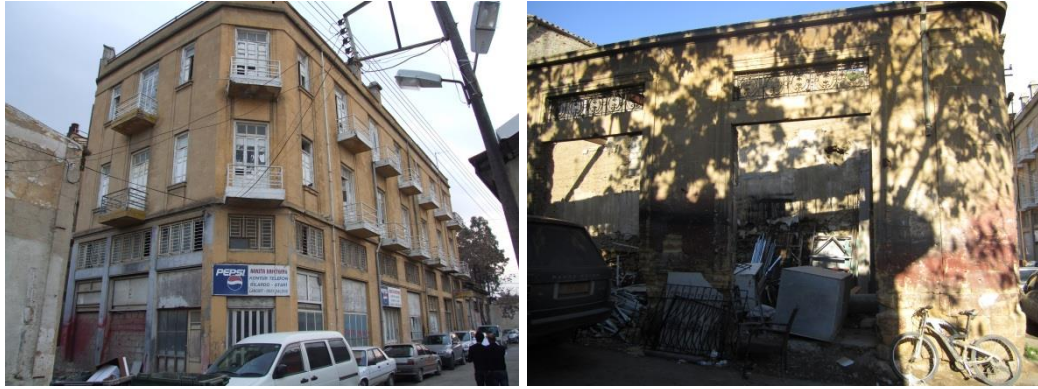
Figure 3. 16. Structural Condition of Buildings in Yediler area (Source: Author)
