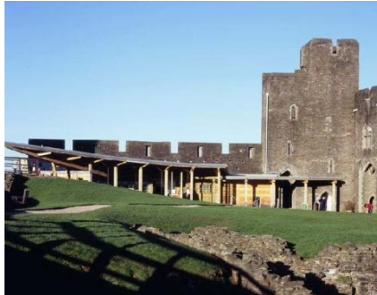
Figure 6: Visitor Centre, Caerphilly Castle, by Davies Sutton
