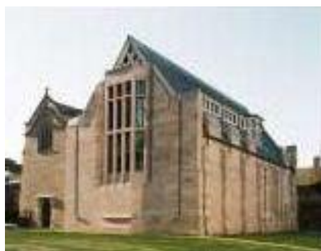
Figure 5: Cathedral Library extension, Hereford, by Whifield Partners (Davies, 2003)
