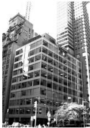
Figure 7: Formerly Pepsico Building (Skidmore, Owings & Merrill, 1960) with office tower addition (right) by James Stewart Polshek and Partners, 1985
