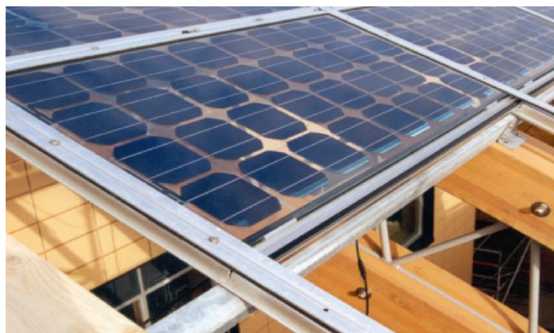
Figure 2.21: Monocrystalline PV in a semitransparent module-glass on the back (Robert and Guariento, 2009, p.27).
