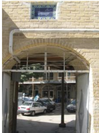
Figure 64 –Entrance of Caravansary from Street (Author, 2012)
