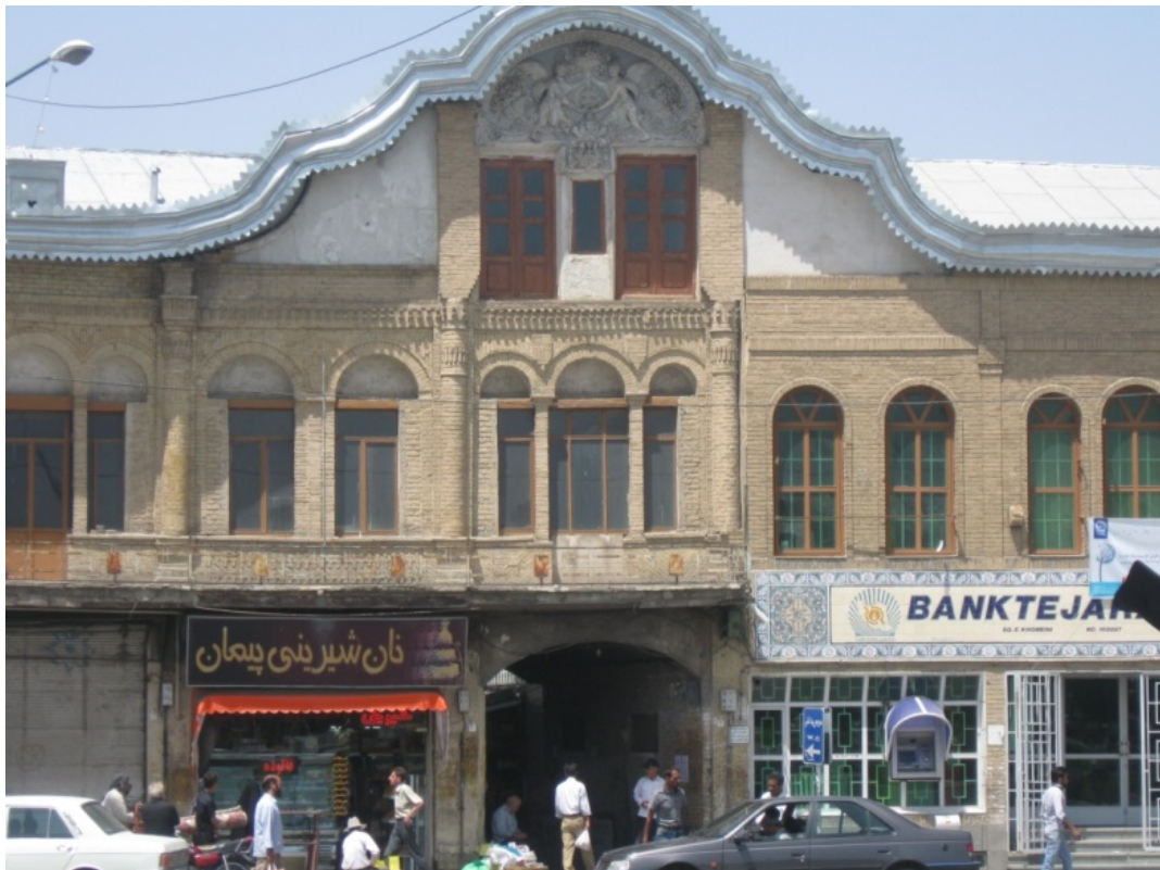
Figure 58 - Entrance of Bazaar from Main Square (Author, 2012)
