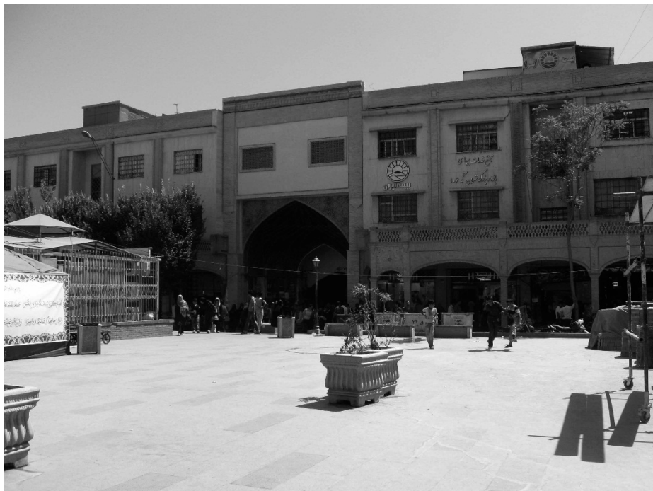
Figure 82 - Main Entrance of Grand Bazaar Tehran (Author, 2012)
