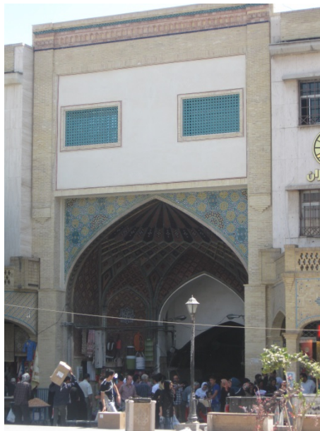
Figure 83- Main Entrance of Grand Bazaar Tehran (Author, 2012)
