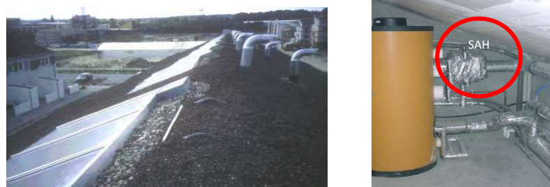
Figure 55: Hannover domestic hot water (DHW), solar hot water storage and supply-air heater (SAH) (Heiduk, 2009)
