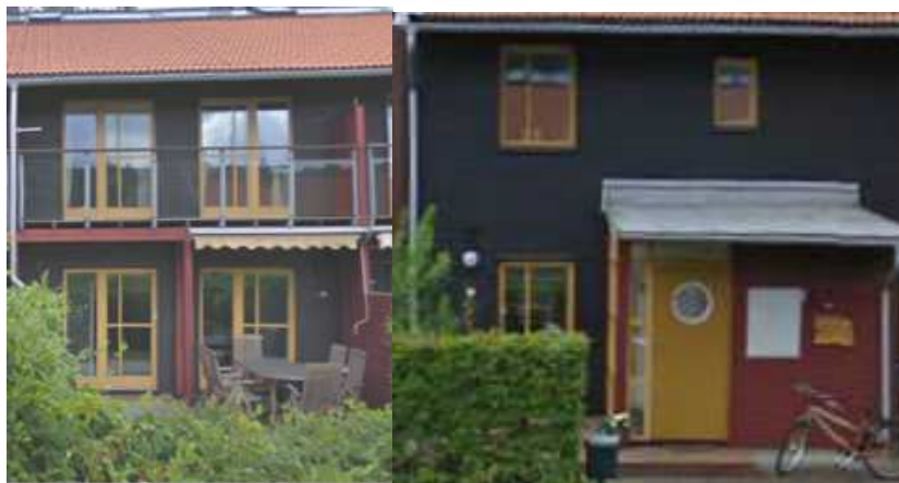
Figure 61: North and south façade windows (Janson, 2009)
