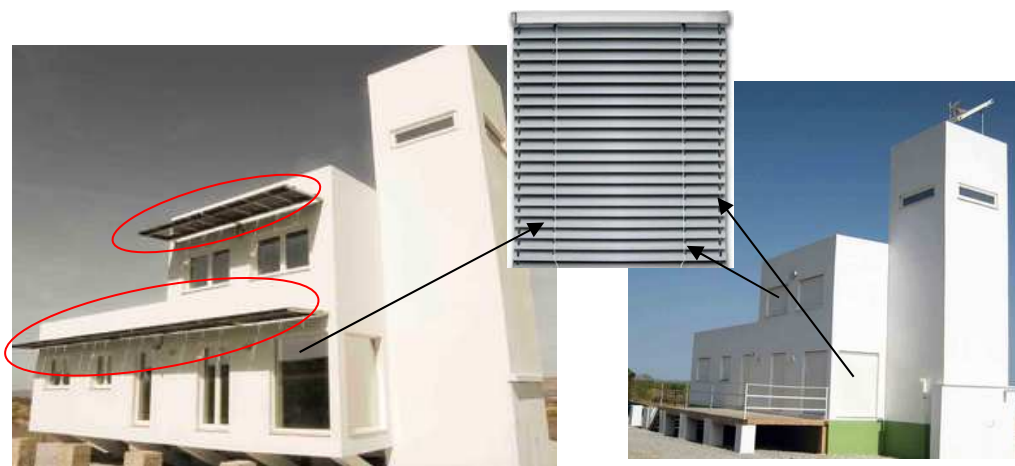
Figure 42: Granada passive house shading device (Construible, 2010)
