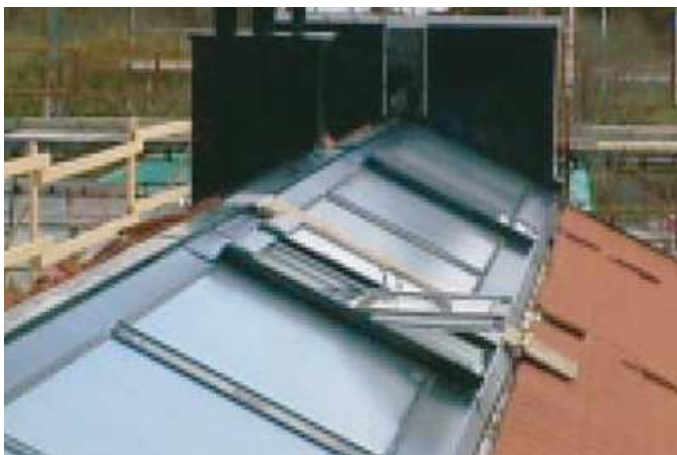
Figure 63: Gothenburg passive house solar collector (Janson, 2009)
