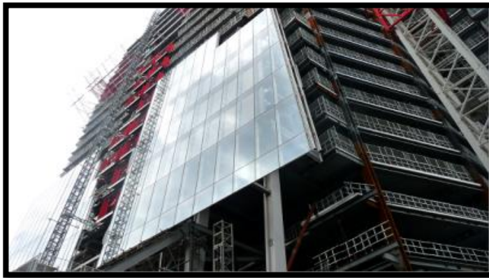
Figure 2.15: Fully Glazed Curtain Walling System Used in a Multi-Story Steel ( www.steelconstruction.facades_interfaces.com )
