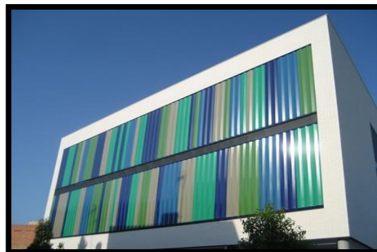
Figure 2.6: Facade of the Library and Cultural Building ( www.thecelosiasofbigshovels.com )
