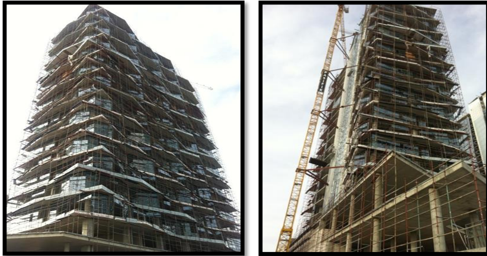
Figure 3.3: Glass Facade with Steel Supporting (Taken by an Author 2013)
