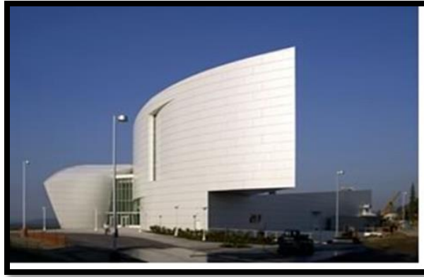
Figure 3.4: Aluminum Cover on the Wall ( www.cmog.com )
