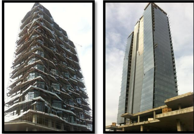
Figure 3.1: The Next level Toki Tower type of Glass with Aluminum Supporting (Taken by an Author 2013).
