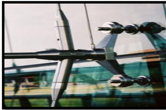
Figure 2.16: Glazing Support System ( www.cmog.org.com )
