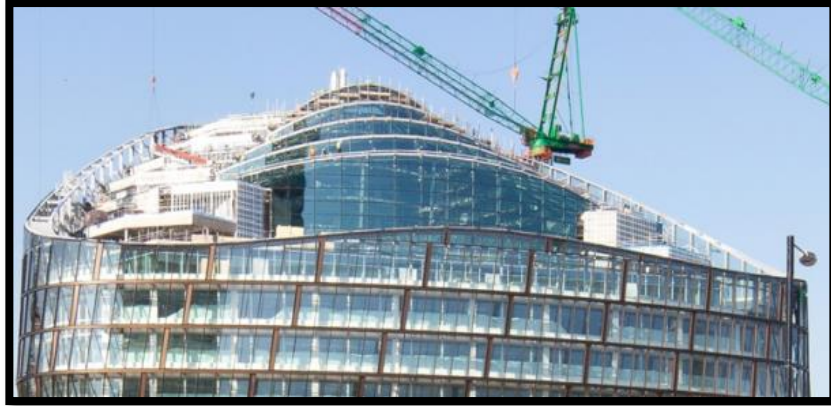
Figure 2.10: Facade Curtain Wall Posses ( http://www.steelconstruction.info/Facades_and_interfaces )
