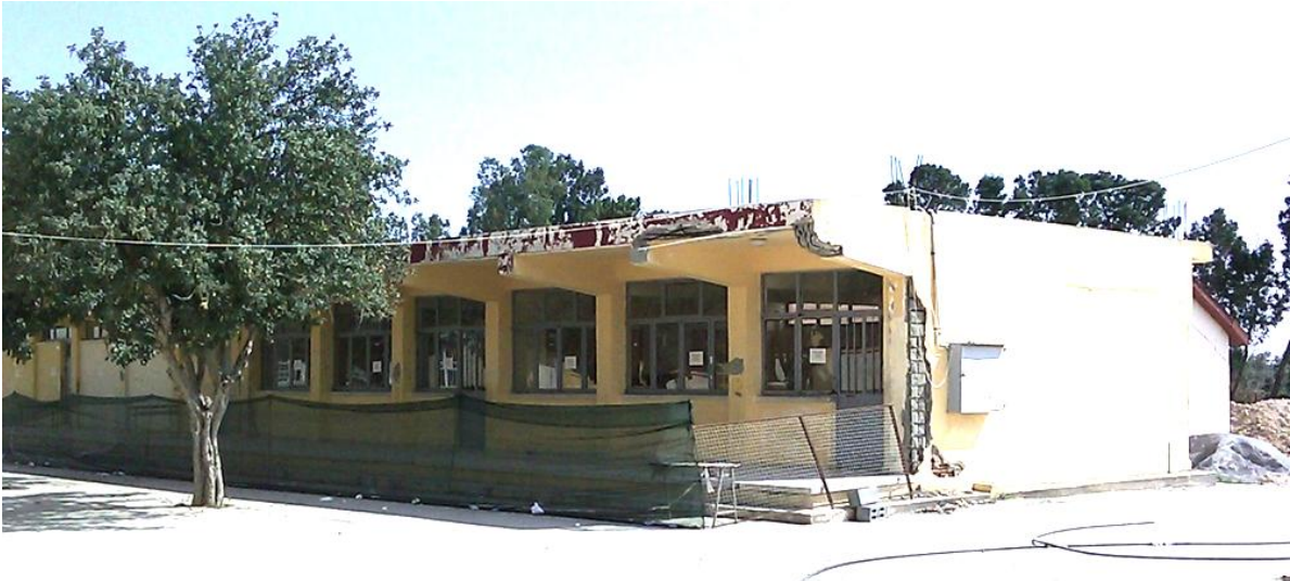
Figure 4.19: Front view of block D
