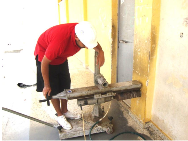
Figure 4.23: Concrete core drilling machine – taking carrot from a column
