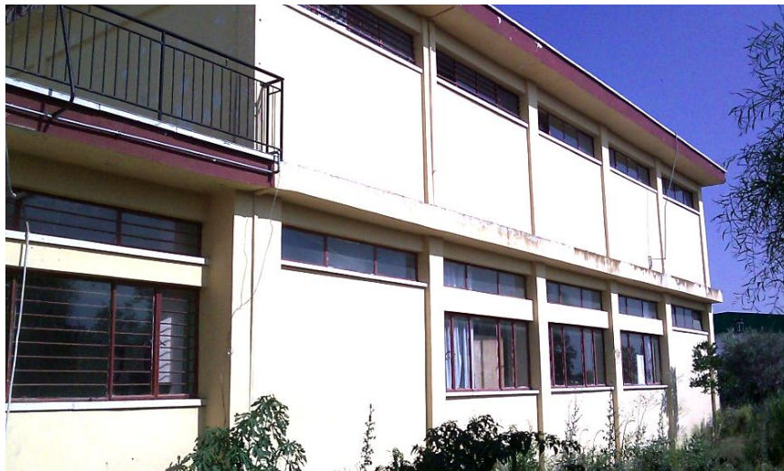
Figure 4.8: Side view of Block B1
