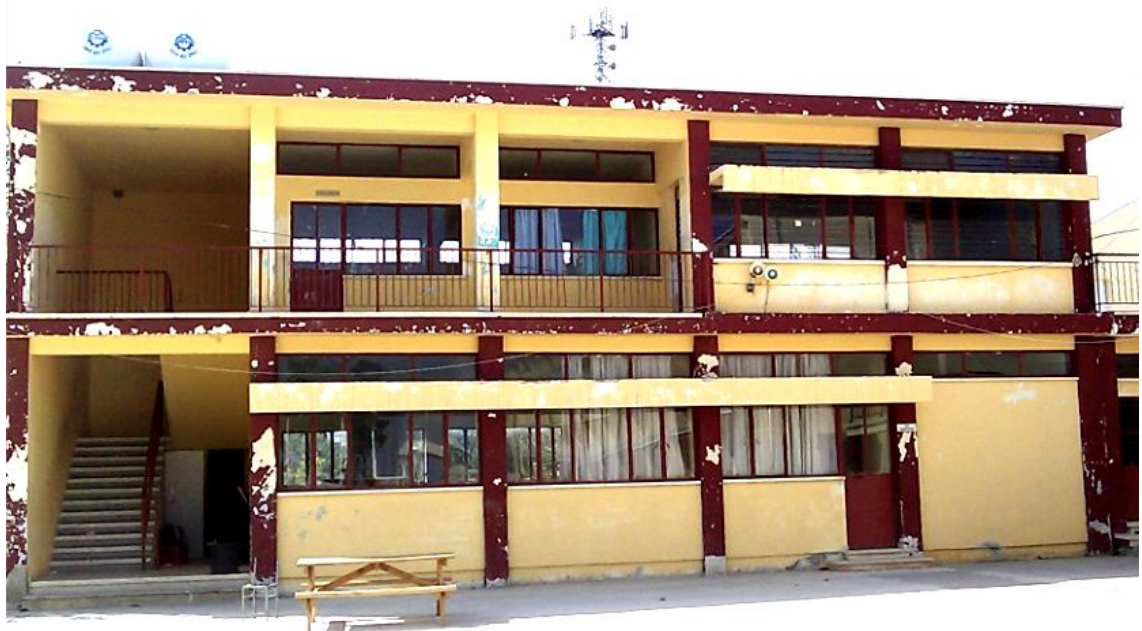
Figure 4.12: Front view of Block B2
