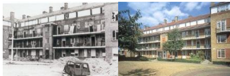
Figure 14: Acorn Walk, Surrey Docks, before refurbishment (left) and after (right) (Source: Monograph archive of The LDDC History Pages, 1981-1998)
