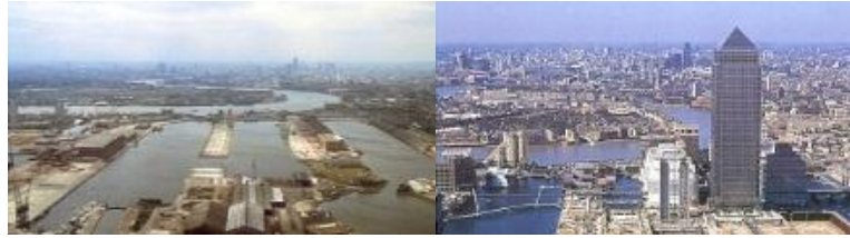
Figure 15: West India Docks, looking west, 1982 (left), Canary Wharf and the Isle of Dogs, 1997(right) (Source: Monograph archive of The LDDC History Pages, 1981-1998)
