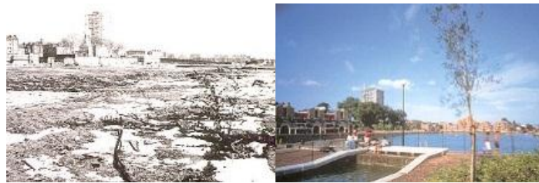
Figure 11: Shadwell Basin 1985 (left), Shadwell Basin 1998 (right) (Source: Monograph archive of The LDDC History Pages, 1981-1998)
