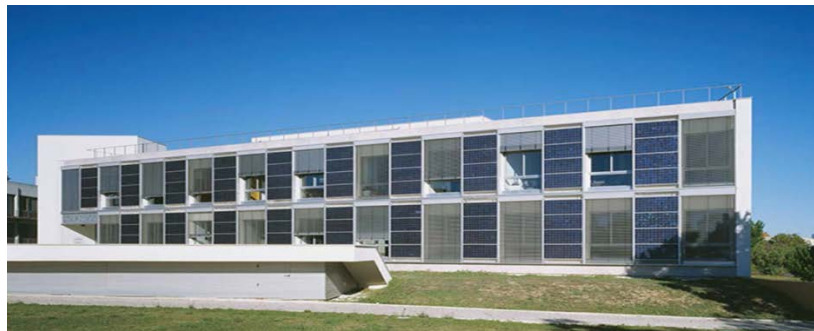
Figure 1.7: PV Integrated into the Opaque Parts of the Façade of Solar XXI Building. (Source: www.enginsolar.com )
