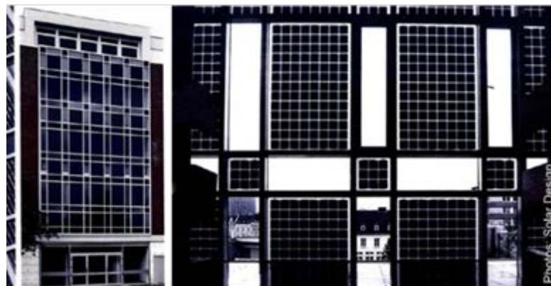
Figure 1.26: One of the First Applications of the Multifunctional Use of PV Systems in the Administrative Building on the Stadtwerke, Aachen, Germany,
