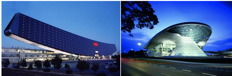
Figure 1.28: Integration of PV, Considering the Formal Aspect. (Left) Solar Ark Japan, (Right) BMW Welt Building in Germany, Architect: Zaha Hadid
