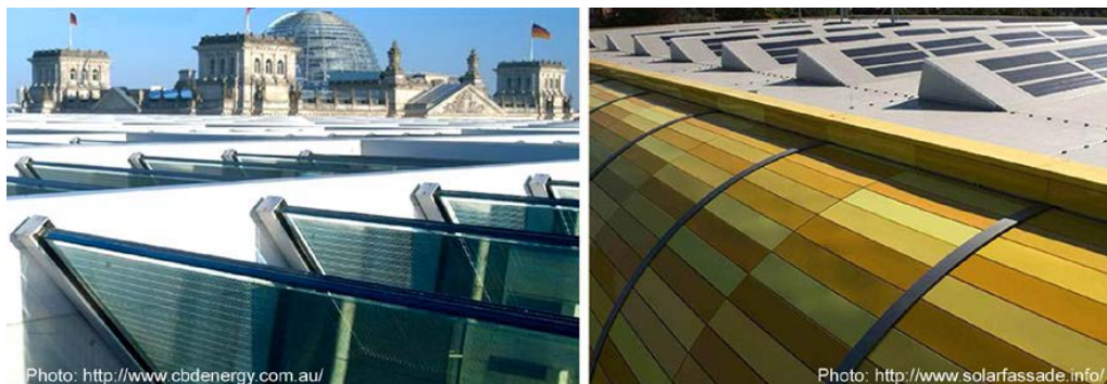
Figure 1.17: (left) Integrated PV on the Saw-Toothed Glass Roof of Paul Lobe Haus, Berlin (right) Saw-Tooth Roof with PV Integration, DIY Store, Hamburg Source: http://www.cbdenery.com.au/ , http://www.solarfassade.info/
