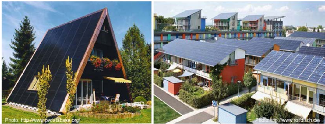
Figure 1.14: (left) Integrated PV on the Pitched Roof of Vacation House Bartholomäuspark in Germany (Right) Integrated PV Roofs in Schlierberg Solar Settlement in Freiburg Source: http://www.pvdatabase.org/ , http://www.rolfdisch.de/
