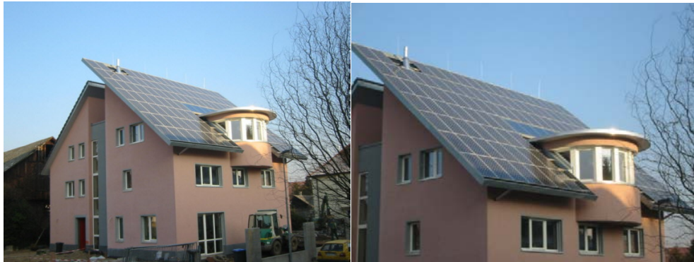
Figure 2.13: Passive House, Emmendingen, Germany. Source: www.enginsolar.com
