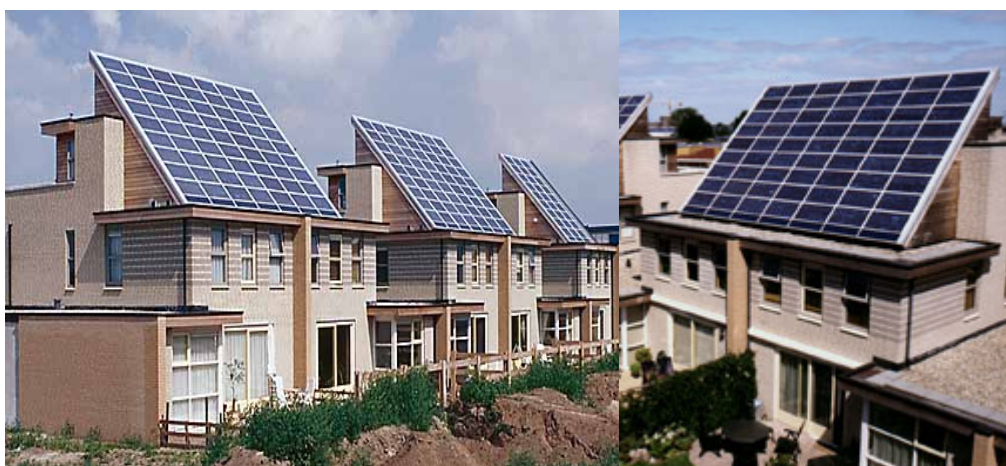
Figure 2.14: Prefabricated PV-Roofs' in Nieuwland District, Amersfoort, Netherlands
