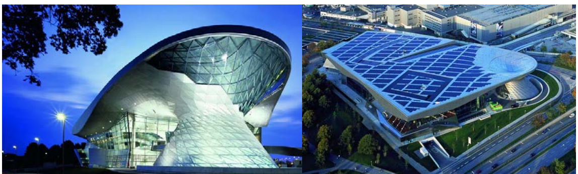
Figure 2.5: BMW Welt Building in München, Germany . (Source: www.enginsolar.com )
