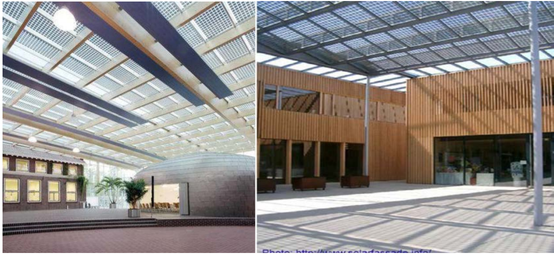
Figure 1.16: (left) Atrium with PV Modules, Ludesch/Voralberg., Austria; (right) PV on Coloured Skylights at Bejar Market, Salamanca, Spain Source: http://www.solarfassade.info/
