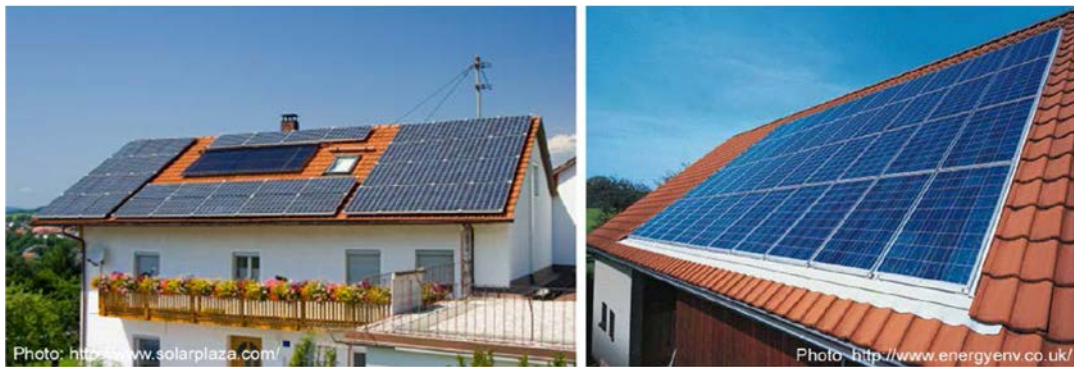
Figure 1.13 (left) PV Modules Added on to the Roof as Pure Technical Element, (right) Semi Integrated PV Modules on the Roof
