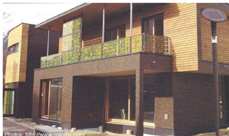
Figure 1.23: PV Modules Based on Metallic Gold Cells are Integrated in the Balcony, Rails and Facade, Tirol, Austria
