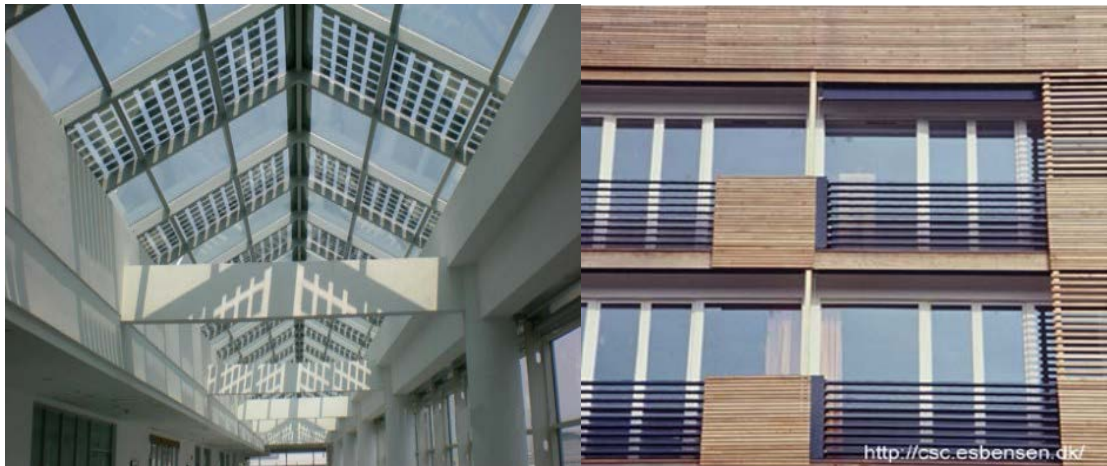
Figure 1.27 (left) Integration of PV as Shading and Daylight Control; (right) Evacuated Tube Collector Used as Balcony Railing
