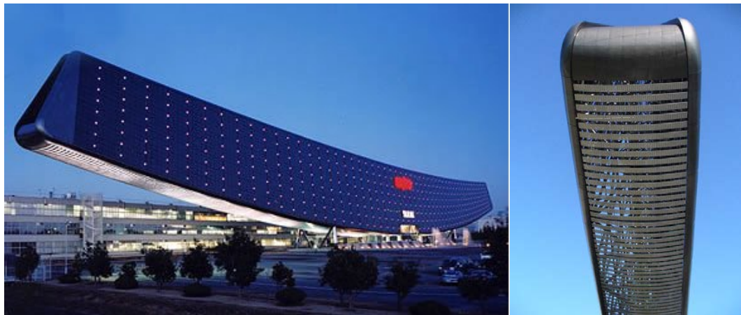
Figure 2.3: Solar Ark Building Ohmori, Japan Source: www.solar.integrateing.com
