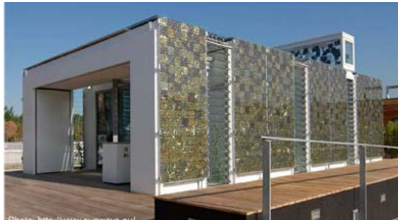
Figure 1.24: Multi-Crystalline PV System with Bronze and Gold Coloured Silicon Solar Cells Used in the "Home+" Building Project Submitted by Stuttgart University of Applied Sciences. Source: Credit: http://www.sunways.eu/
