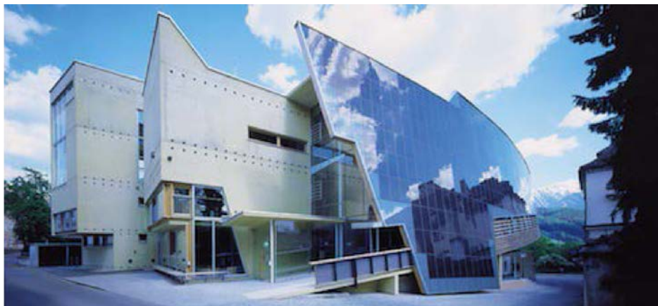
Figure 1.10: Inclined PV Integrated Glazed Façade of Vocational College in Tirol, Austria. Source: http://www.m9-architekten.at/
