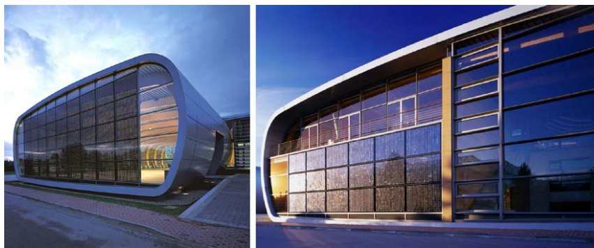
Figure 1.8: PV Integrated into the Opaque Parts of the Façade of Solar in Germany. (Source www.enginsolar.com )
