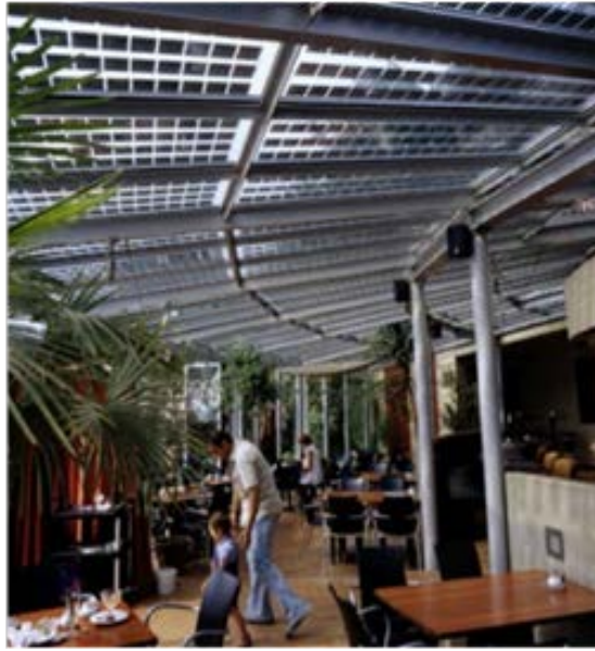
Figure 1.12: PV Integrated Double Glazed Roof of Café Ambiente, Berlin Germany Source http://www.pvdatabase.org/
