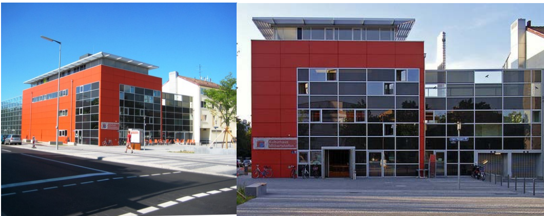
Figure 2.6: Cultural Centre in Milbertshofen, Germany Source: www.enginsolar.com
