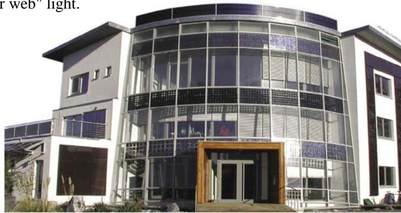
There are 11 solar systems integrated on, in and on top of the office building of Centrosolar AG (Paderborn/Germany location)
