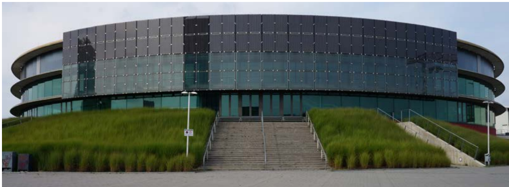
Figure 2.1: EWE Arena, Oldenburg, Germany. Source http://www.iea-shc.org/
