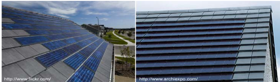
Figure 1.15: Integrated PV Roof Tiles on the Roof in Berlin Germany
