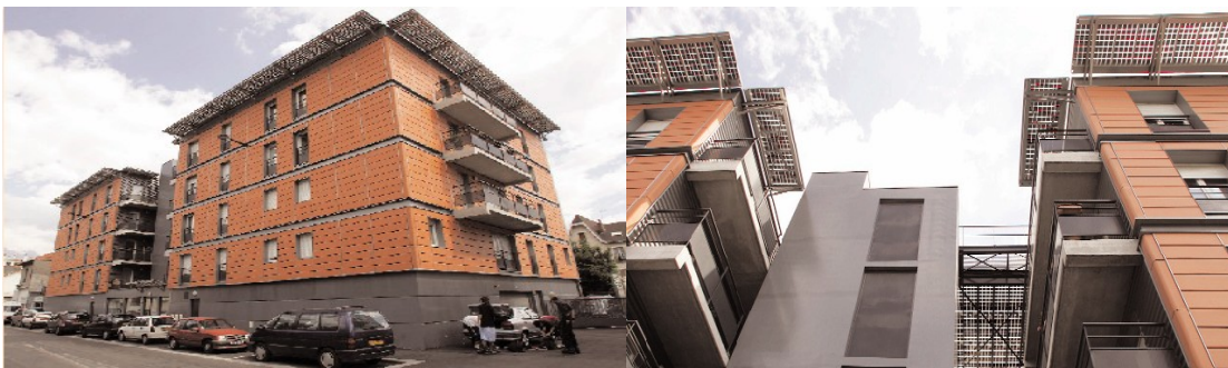
Figure 2.17 Social Housing Moyrand Street (22 kWp), Grenoble, France Source: www.enginsolar.com
