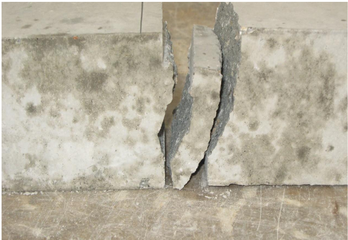
Figure 69: Shear cracking in plain concrete
