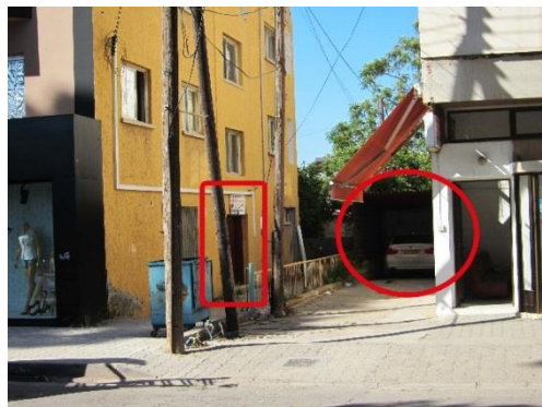
Figure 3.17: Example of Combination of Building Entrance and Parking Entrance Contribute to the Increase of Surfaces More Than Two (Photo taken by author)
