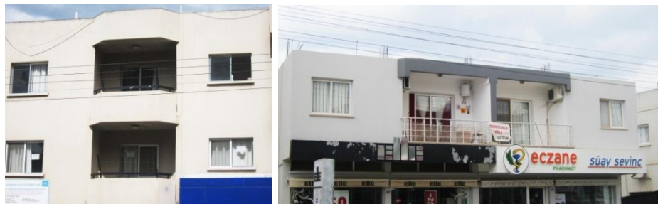
Figure 3.20: Examples of Loggias Which Are Shaded Building in Southwest Direction (Photos taken by author)
