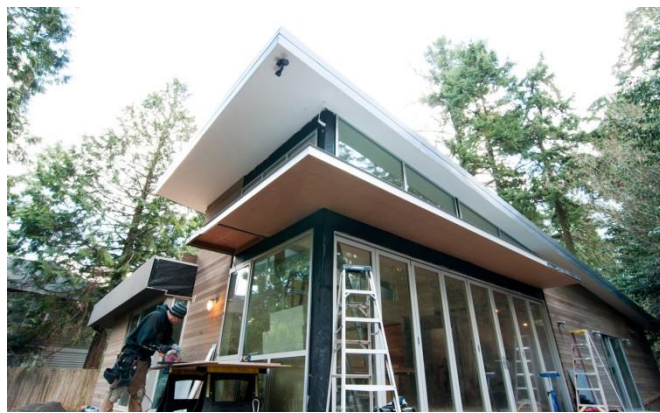
Figure 2.27: Example of Light Shelf Overhang. Illustration taken from blog.buildllc.com
