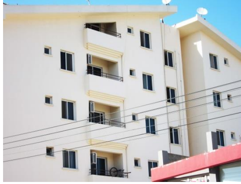
Figure 3.22: Example of Loggias Which Are Shaded Building in Southeast Direction (10% of Openings) (Photo taken by author)
