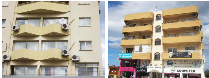
Figure 3.23: Example of Balconies Which Are Shaded Building Horizontally (Photos taken by author)
