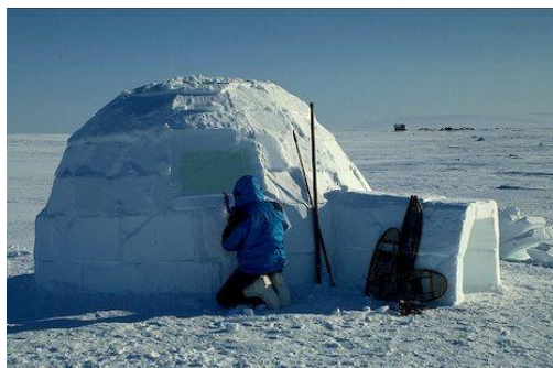
Figure 2.10: An Igloo Has a Suitable A/V -Ratio (Illustration taken from URL: http://www.montserratvolcano.org/merapi%202.htm )
