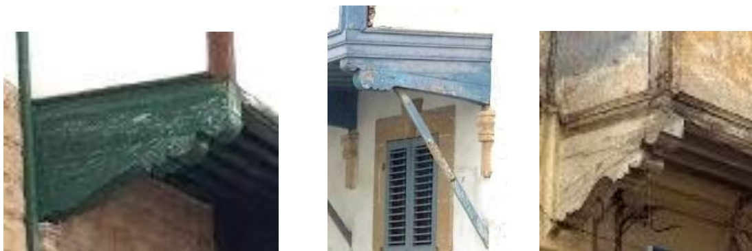
Figure 31 & Figure 32 & Figure 33: Three Common Types of Brackets in Cyprus Houses Facade
