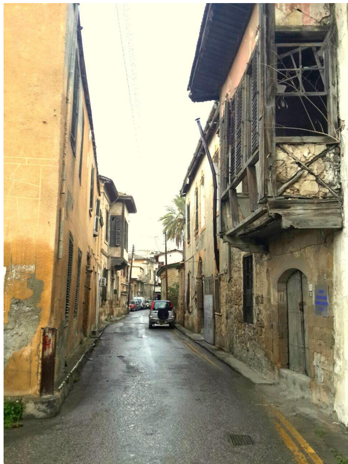
Figure 18: Ottoman Street Was Shaped with Houses (Wall-City, Nicosia)
