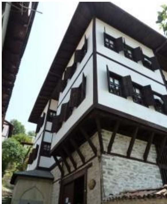
Figure 28: Windows' Shutters in Ottoman House (URL14)
