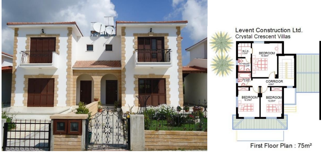
Figure 58: Second House Image (Crystal Crescent– Bogaz Village, Girne)
