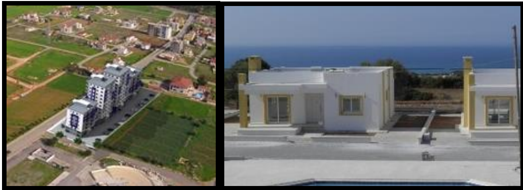
Figure 78 & Figure 79: Park View Towers in Yeniboğaziçi Village and Port Karpaz in karpaz, Famagusta
