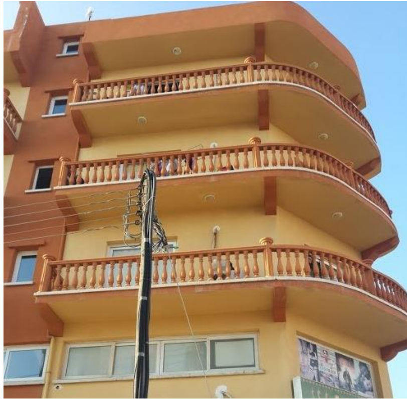
Figure 56: Wide Balconies in Front of the Contemporary Residential Building (Famagusta)
