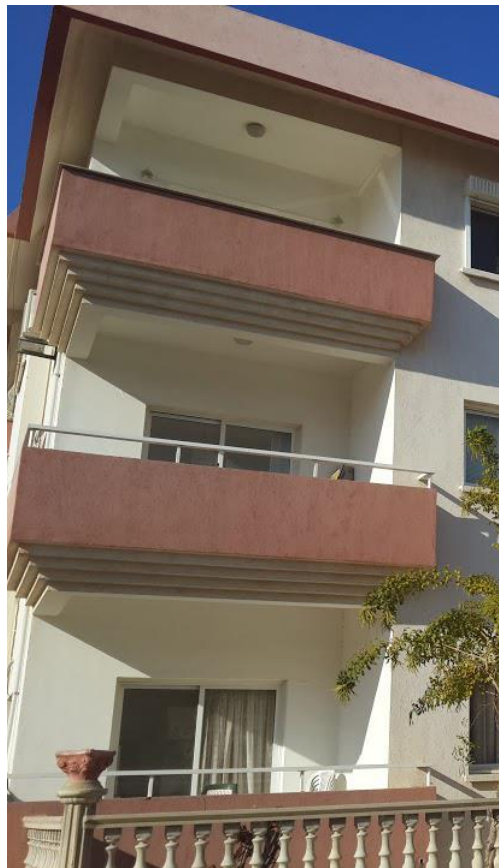
Figure 55: Symbolic Use of Brackets in Contemporary House (Famagusta)
