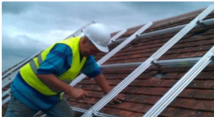
Figure 3.119: Mounting the Profile Carriers of the Panels on the Roof Surface
