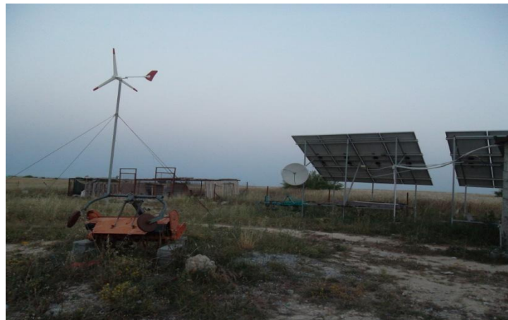
Figure 3.61: Photo shows Wind Tribune and 12 Poly-crystalline Panels (Taken by author)
