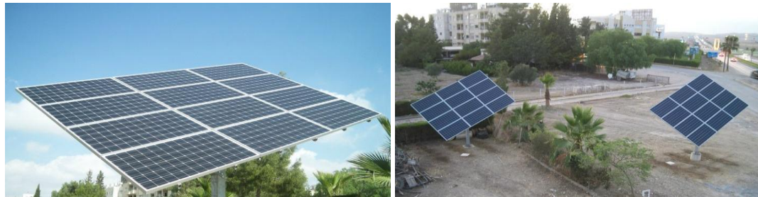
Figure 3.19: Photos are showing 24 Mono-crystalline Cell Type Panels on 2 Single-axis Sun-tracker System (Ekrem Güneş Solar, 2013)
