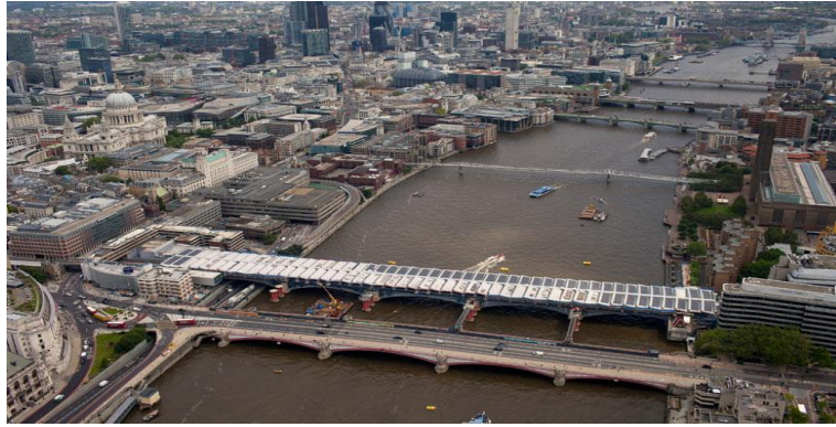
Figure 3.111: General View of the Station with the Photovoltaic Arrays (Solar century, 2013)
