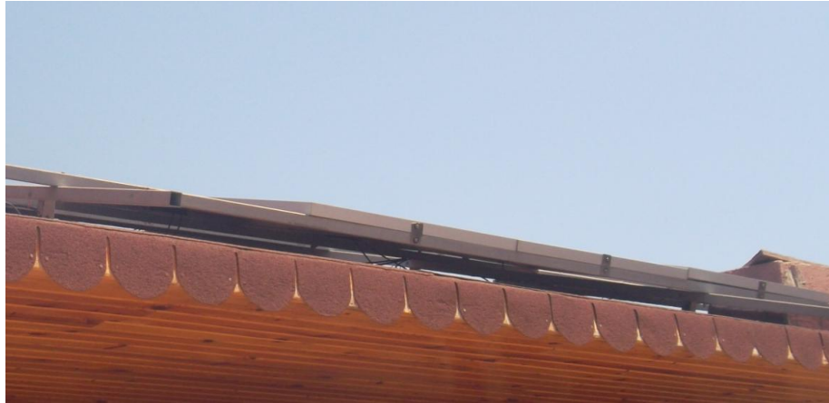
Figure 3.69: Distance between the Panels and the Roof Surface (Taken by author)
