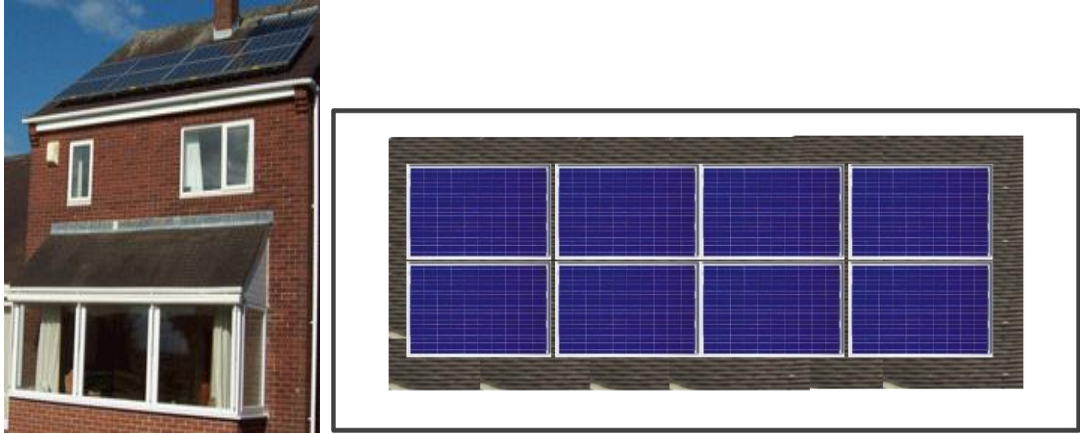
Figure 3.126: Photo shows the 3 rd House Panel and the Top View (Landscape Organization)
