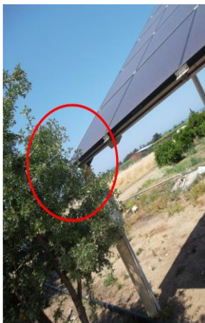
Figure 3.4: Trees Shading Panels (Photo Left) and the Space between the Panels and Supporting Element (Photo right) (Taken by author)
