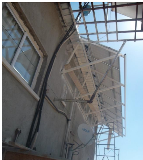
Figure 3.77: Photo shows how Panels Supported (Taken by author)
