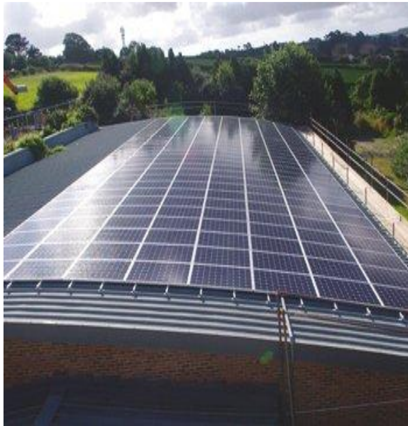
Figure 3.107: Photo shows the General View of the Panels (Sambata, 2012)
