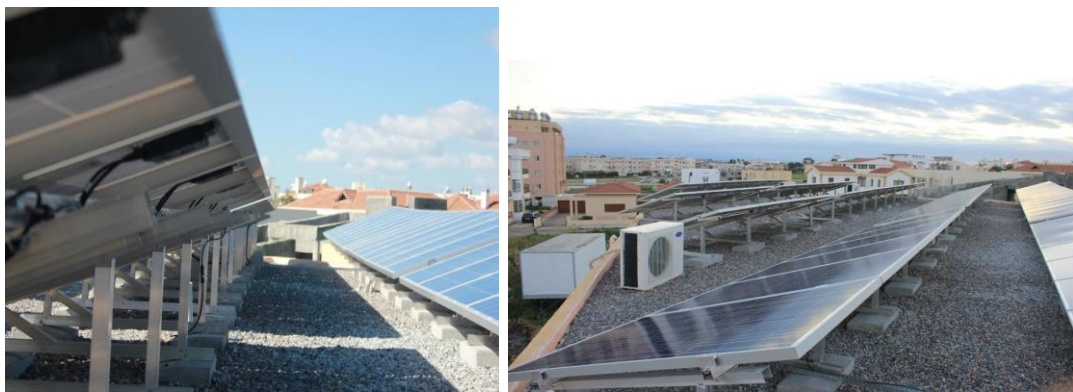
Figure 3.40: Photos show the Distance Between the Two Arrays (Ekrem Güneş Solar, 2013)
