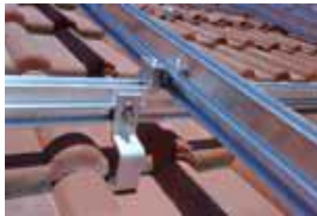
Figure 3.30: Connection Detail of the Support (Brooks, Dunlop, 2012)
