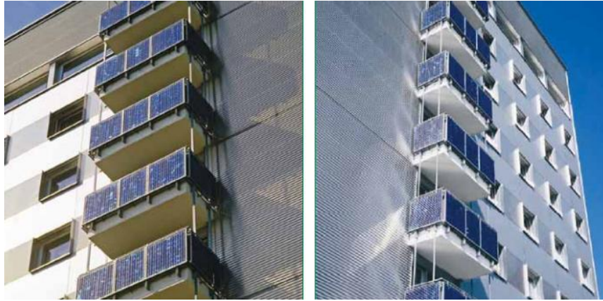
Figure 2.20: Example for PV Integration as a Balustrade
