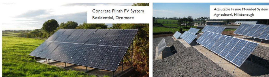
Figure 2.19: Photos show the Freestanding Examples Supported by Profile Carriers (Horizon Renewables, 2013)
