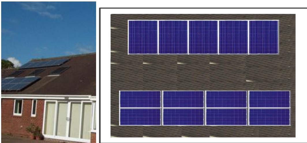
Figure 3.125: Photo shows the 2 nd House Panel and the Top View (Portrait and Landscape Organization)
