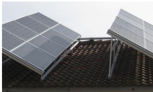
Figure 2.25: Shading from front panel (Self shading)
