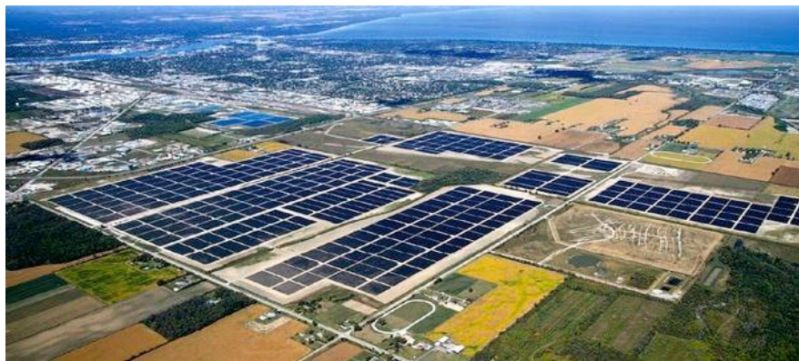
Figure 3.92: Top View of Power Plant (Enbridge, 2010)
