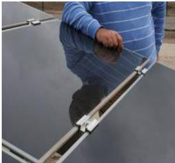
Figure 3.99: Thin-film PV Modules at Templin Solar Park (Schwers, 2012)
