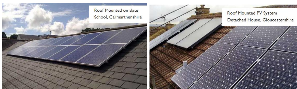
Figure 2.11: On-roof Location Type Applications (Horizon Renewables, 2013)
