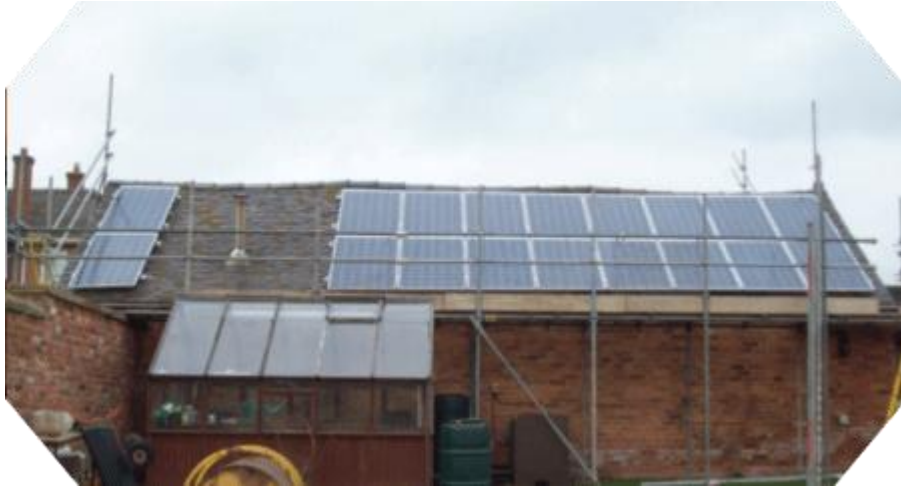
Figure 3.142: View of the Front Building with the Panels
