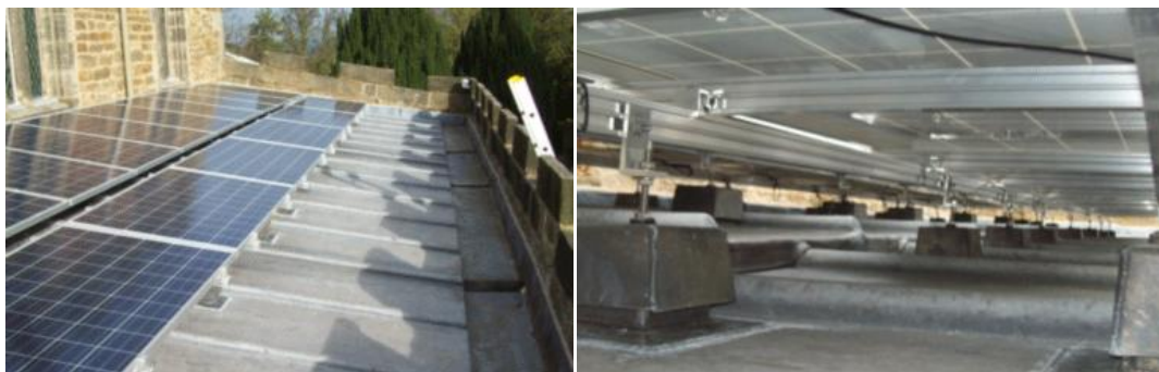
Figure 3.146: General View of the Panels Installed to the Façade of Building
