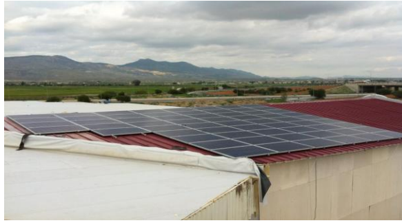
Figure 3.57: Poly-crystalline Cell Type Panels on the Metal Sheet Roof (Ekrem Gunes Solar, 2013)
