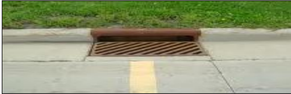
Figure 4.1: Typical Inlet Structure
