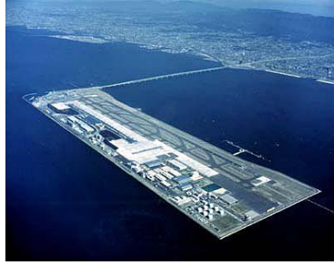
Figure 76: The artificial island and the bridge
