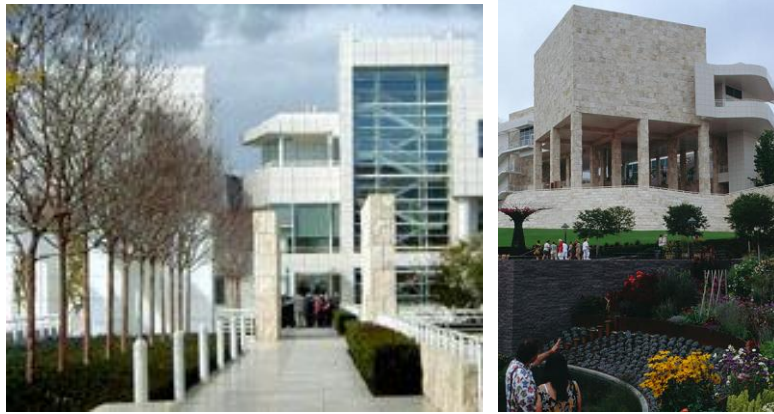
Figure 40: Views of the buildings showing the usage of travertine and white marble
