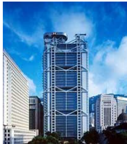
Figure 26: Building showing exoskeleton trusses
