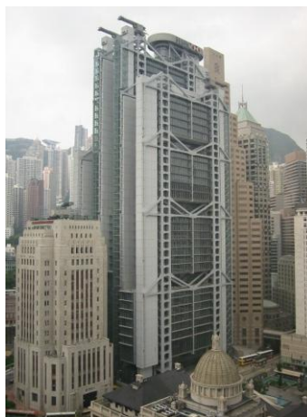
Figure 30: Two metal rods towards the Bank of China Tower
