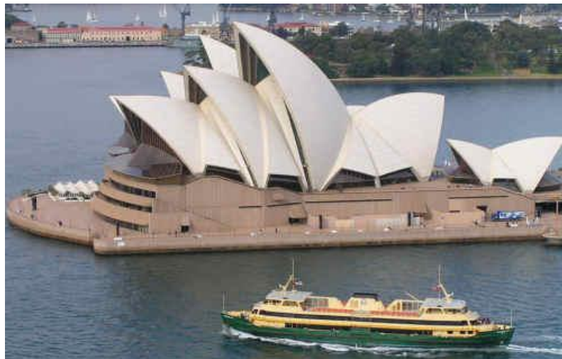
Figure 72: The situation of the Sydney Opera House
