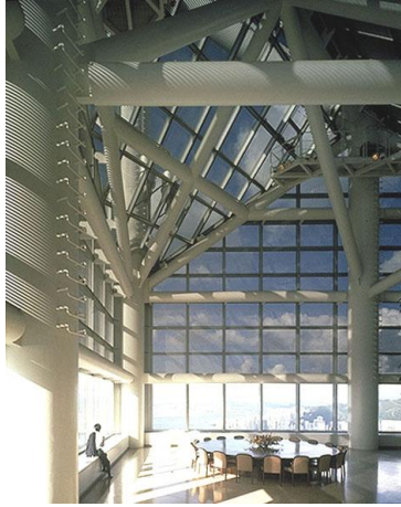
Figure 33: Interior showing the innovative structural system
