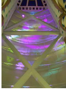
Figure 53: Translucent white fabric stretched around the structural frame
