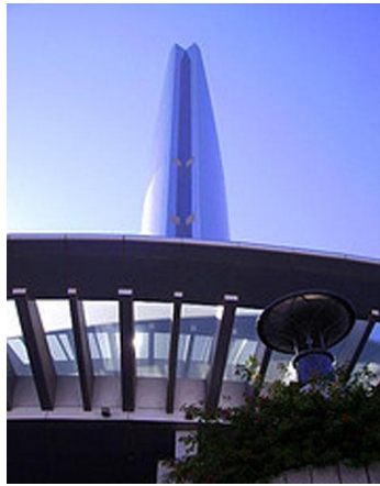
Figure 65: One of the entrances
