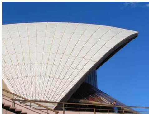
Figure 70: Glazed white granite roofs
