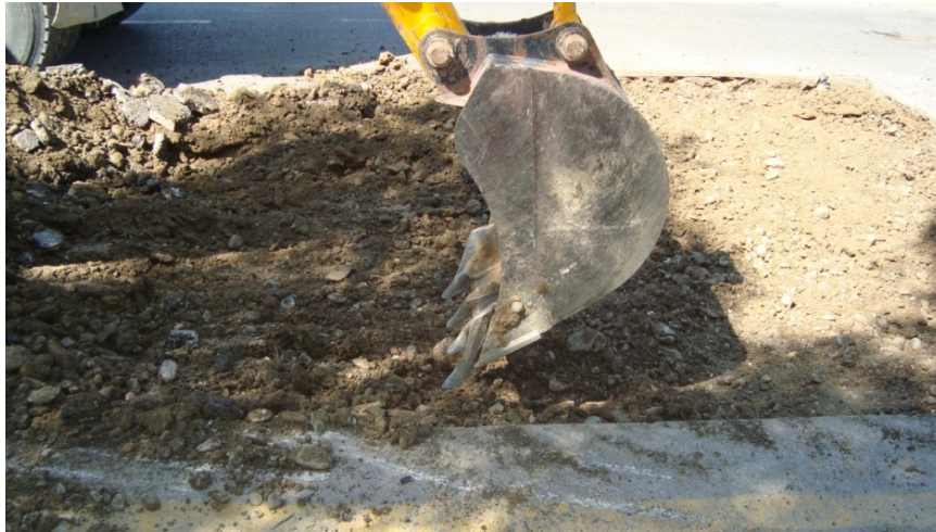
Figure 1.1:Excavating base of selected area.
