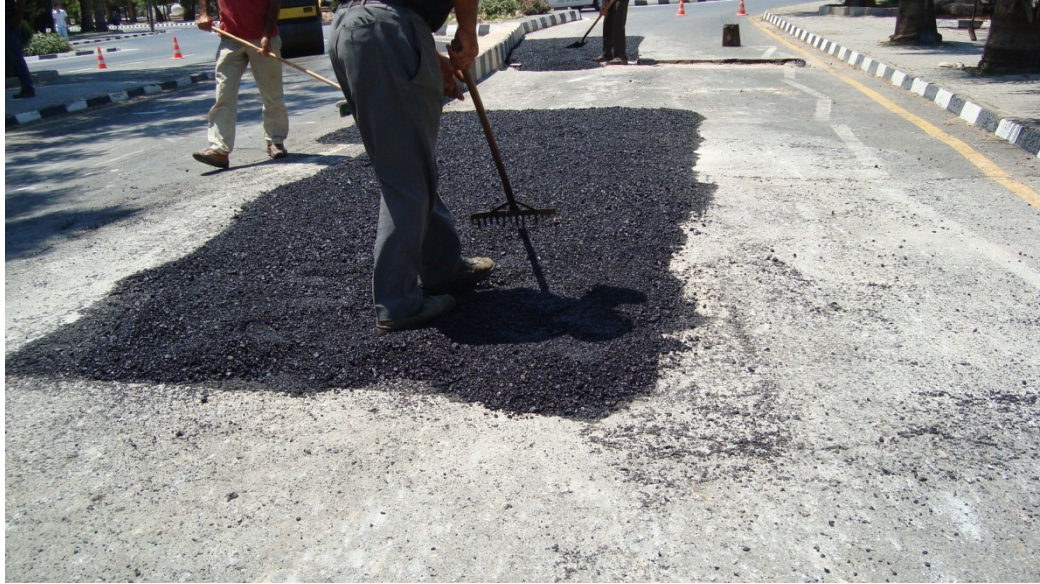
Figure 1.4: Patching work.
