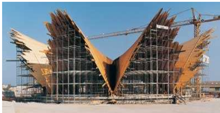
Picture 9: Examples of Concrete thin shell by Felix Candela, Spain [ http://www.greatbuildings.com ]
