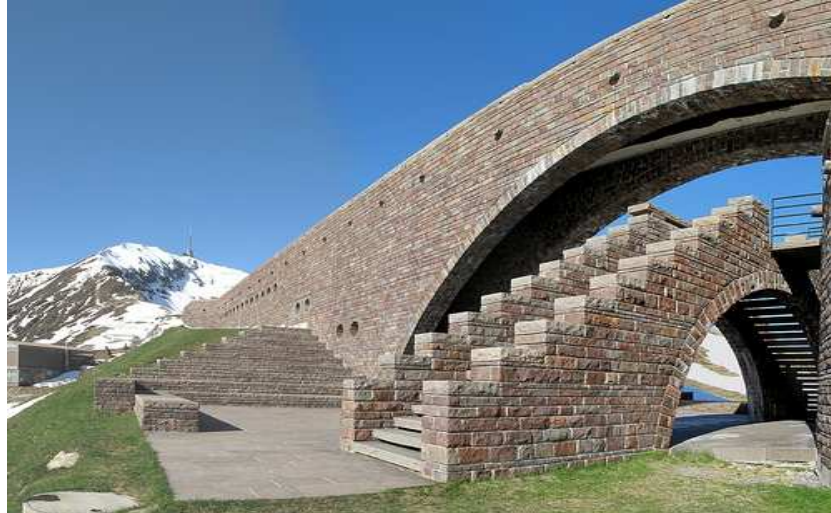
Picture 43: Detailed view for the stone cladding on the walls [ http://www.botta.ch/Architecture/Sa%201996_188.jpg ]
