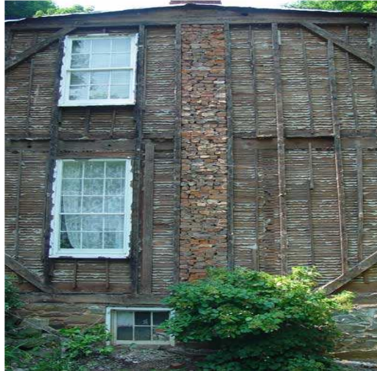
Picture 45: The picture of Balloon Framed timber building [ http://www.hereandthere.org/oldhouse/balloon-framing.html ]
