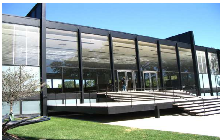
Picture 49: Mies Van Der Rohe's the illinois Institute of Technology in Chicago at 1940 [ http://architecturerevied.blogspot.com ]
