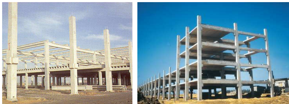
Picture 34: Post-beam structure frame system photos [ http://www.column&beamstructures.com ]
