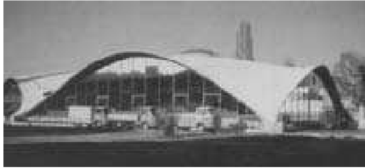
Picture 10: Example of R.C. thin shell which is made by architect Heinz Isler, 1969, Spain [Chilton, p.121, 2000]
