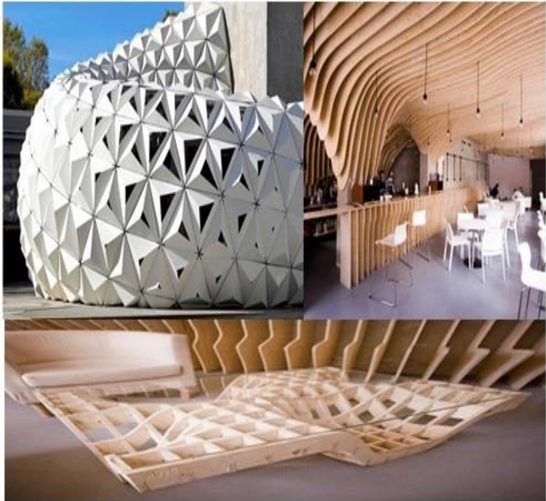
Figure 16: CNC milling, Left: Shell structure by Stuttgart University, Right: Zmianatematu café by Polish architects Source: (Halbe, 2013).
