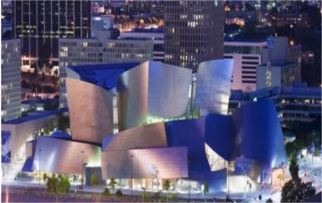
Figure 17: CNC Welding walt-disney-concert-hall, Los Angeles architect, Gehry Source: (Liz, 2007).
