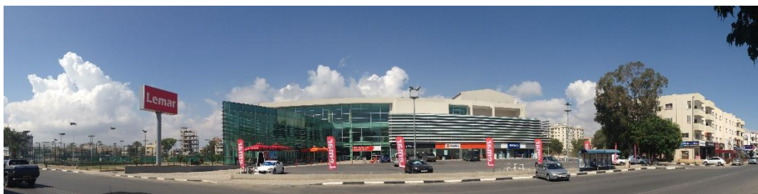
Figure 82: Lemar Complex as a mixed-use building
