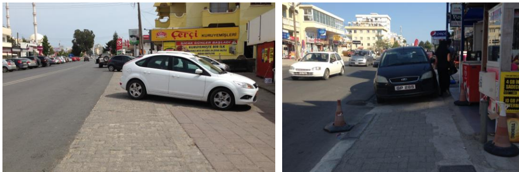
Figure 63: Blocked sidewalks with cars
