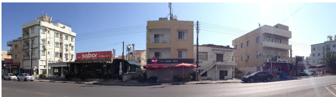
Figure 47: Irregularity in building height and advertising of ground floor
