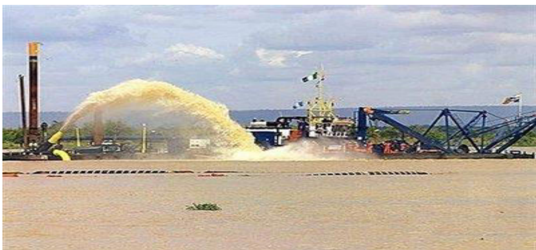
Figure 3.1: Dredging work at Lokoja (Source: AFP, 2009)
