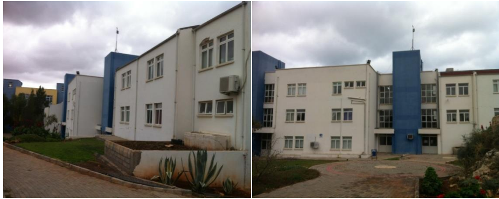
Figure 6.5: South West Façade is Exposed to Direct Solar Radiation (By Author)
