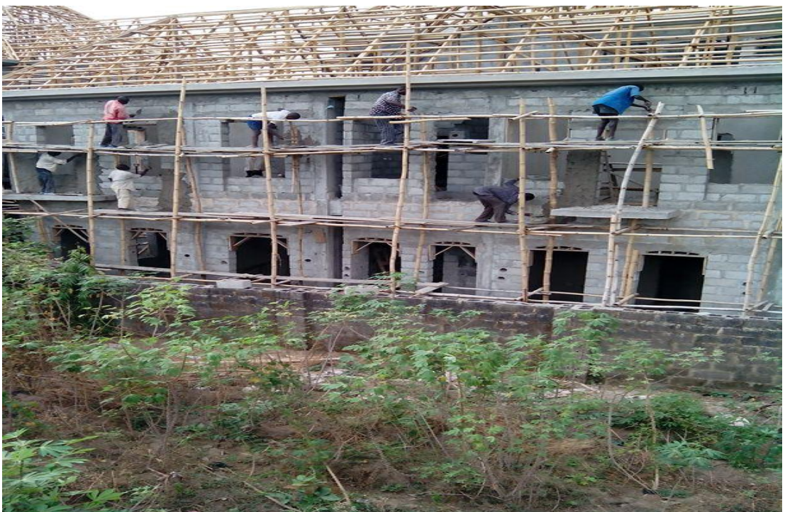
Masons and Labourers working at height without personal protective equipments
