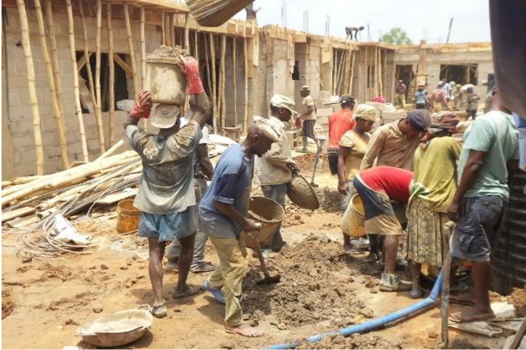
Worker mixing cement bare footed on site
