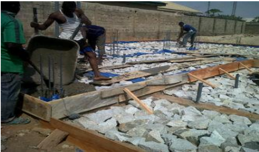
Worker working bare footed on site
