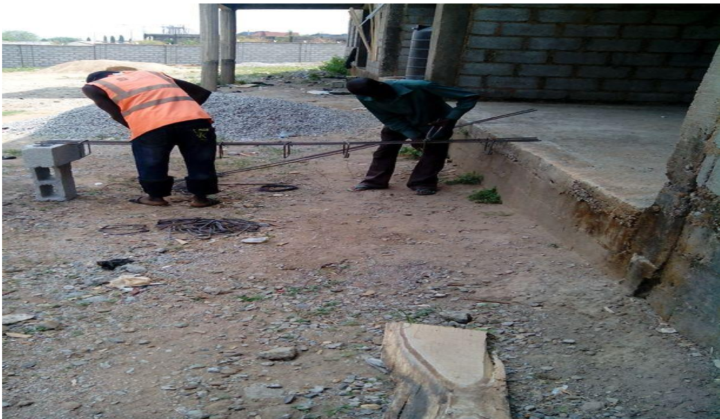
Steel Benders working on reinforcement bars without hand gloves, boots or Helmets
