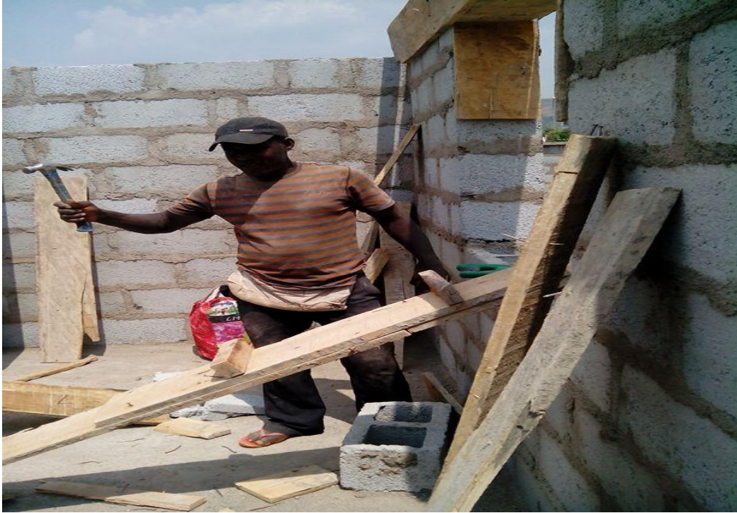
Carpenter creating formworks without hand gloves
