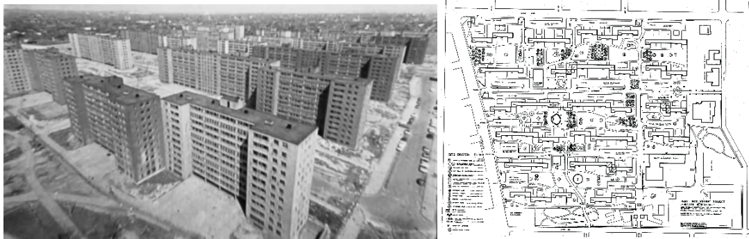
Figure 2.7. The project of Pruitt-Igoe ( http://www.imdb.com ).
