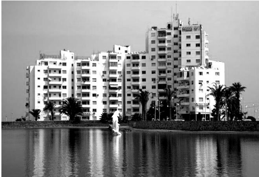
Figure 4.3. Laguna Apartments, western front, (URL2).
