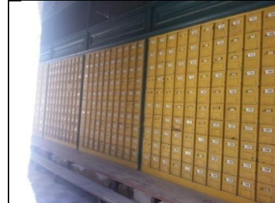
View from outside showing Post Office mail boxes on the ground floor
