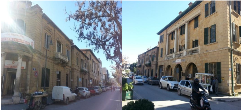
Figure 4.7: Photograph showing street scape views from outside the Colonial Post Office Nicosia, North Cyprus with other nearby historic heritage buildings. (Author, 2014)
