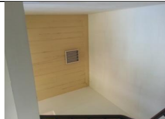
View from inside the Post Office building showing the wooden ceiling
