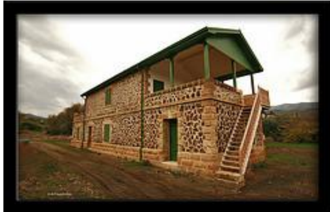
Figure 3.26: Restored Colonial railway building in Evrychou Nicosia, Cyprus. (URL 18)
