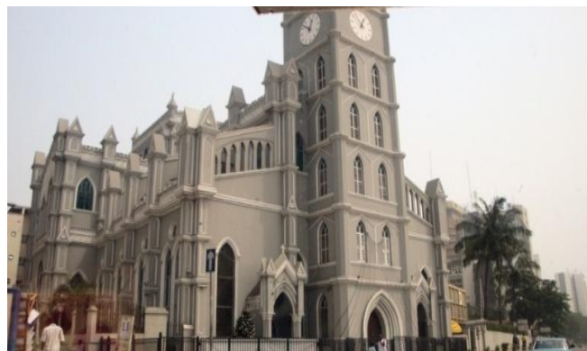
Figure 3.19: Cms Church Lagos, Nigeria. (URL 16)
