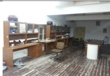
Photo showing wooden floor in basement
