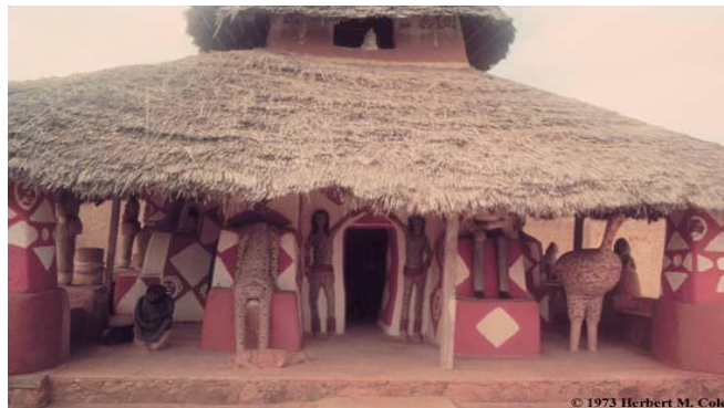
Figure 3.5: Picture showing the elaborate Mbari decorations in traditional Igbo architecture. (URL 6)
