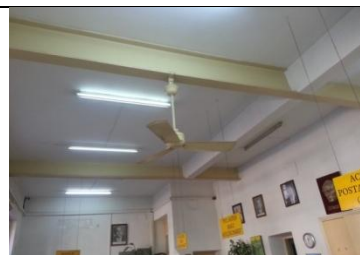
View showing the wooden upper floor been supported by beams
