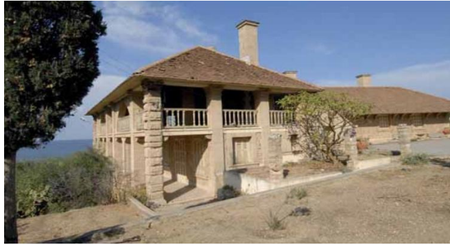
Figure 3.30: Latomia Caroes house, Kyrenia. Built in 1933. (Cyprus Today, 2013)
