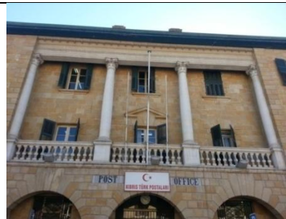
Photo showing Tuscan columns synonymous to British Colonial Period.
