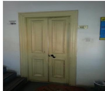
Historic door on ground floor leading to (stair case area)
