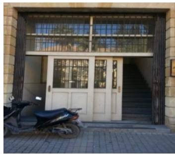
Side entrance leading to basement and top floors
