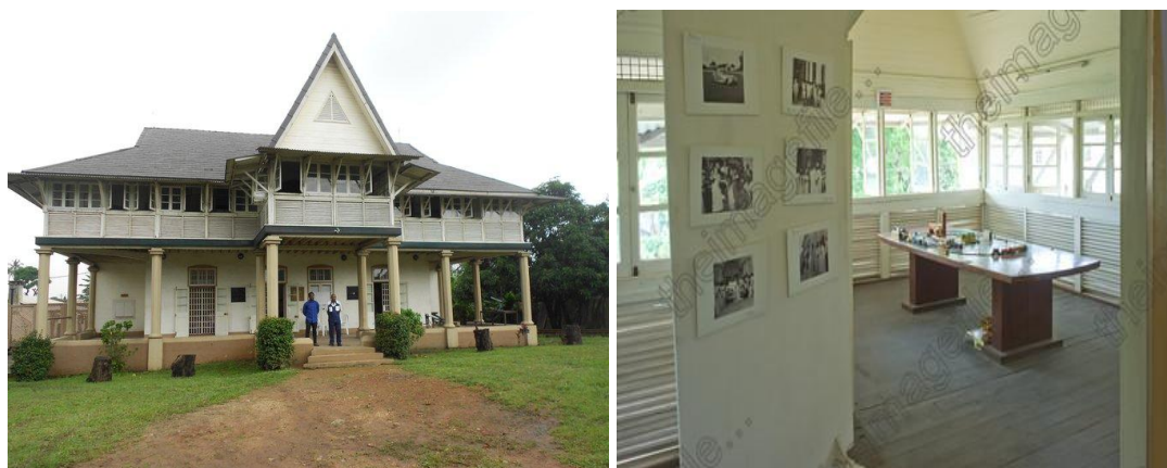
Figure 3.16: Approach and interior of Jakeal House at Lagos, Nigeria. (URL 13)
