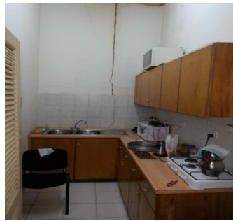
Kitchen to Post Office building on the second floor
