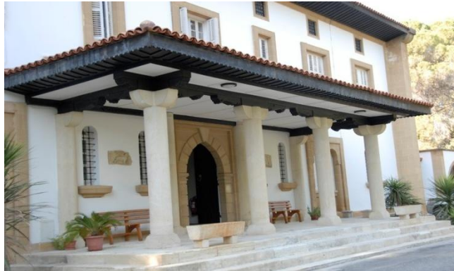
Figure 3.28: British high Commissioners Residence Nicosia, built 1933. (URL 20)
