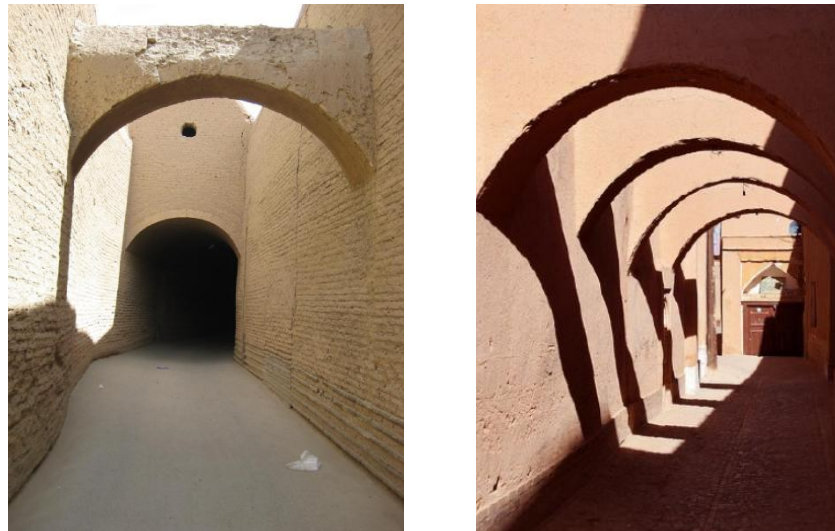
Figure 25: Covered Street in Yazd, a Sabaat in Yazd
