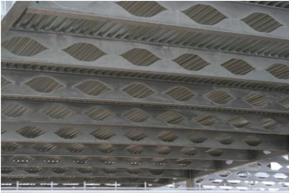
Figure 3 Angelina beams with sinusoidal openings ( ArcelorMittal, 1996 )
