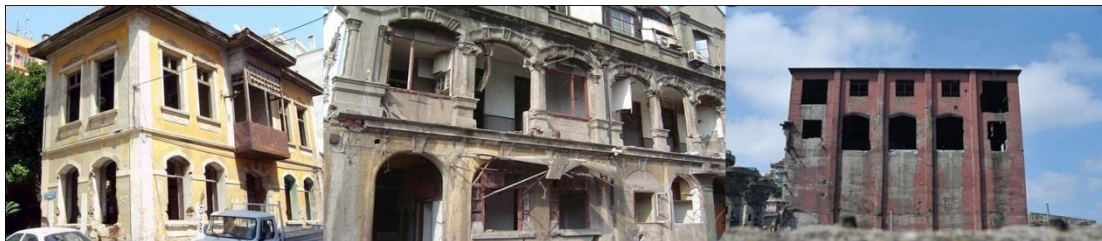
Figure 17: Unused Existing building stocks Source: www.takiplen.com
