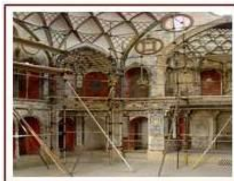
Figure 18. Broujerdiha's hall (Talar) in Kashan. Photo by: Roham Sheikholeslami (URL 9)
