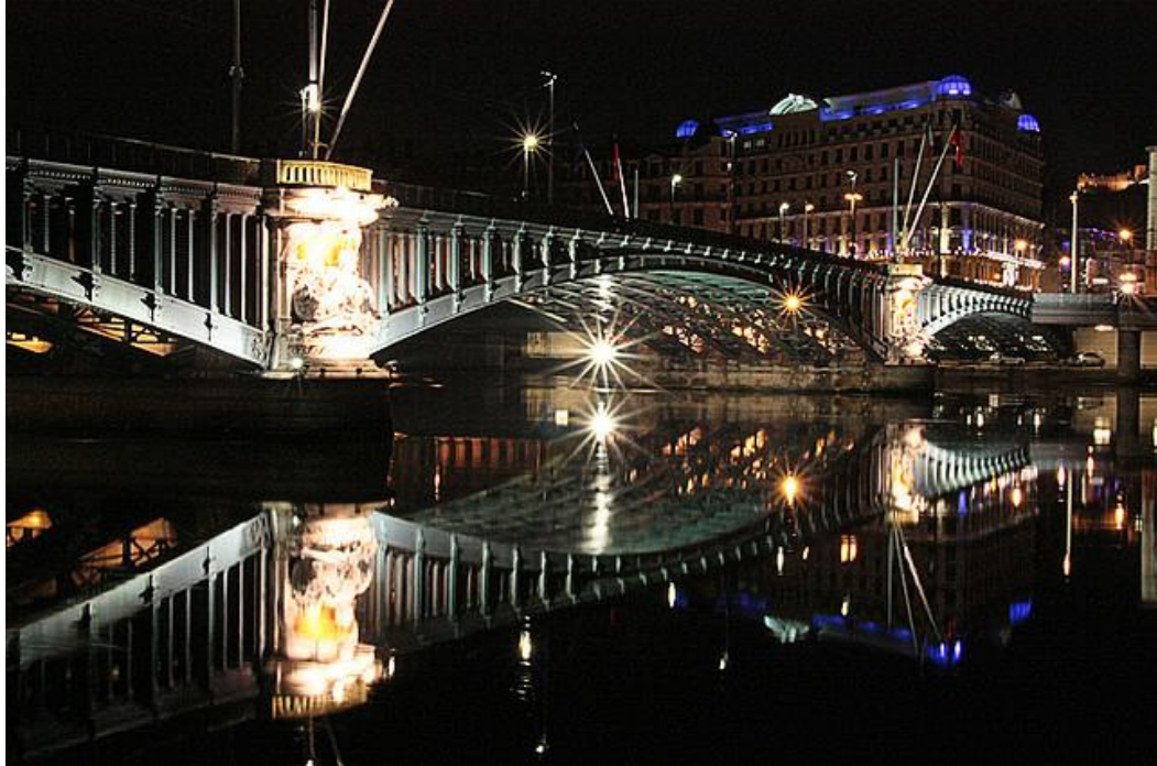
Figure 33: Bridge lighting in Lyon
