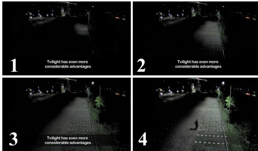
Figure 10: Intelligent street lighting proposed by TU Delft saves up to 80% energy
