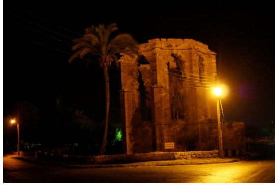
Figure 62: High mounted street lamp causes glare effect in front of high historical building. (Photo by Author)
