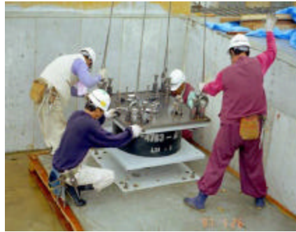
Figure 4.5: Installation of the isolator (Dogan, 2007).
