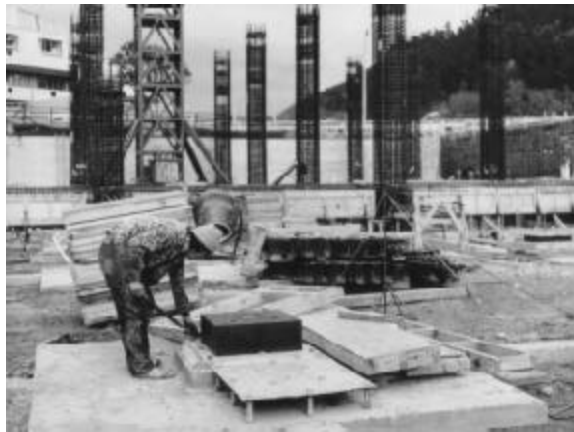
Figure 3.1: Wellington Clayton Building during construction.
