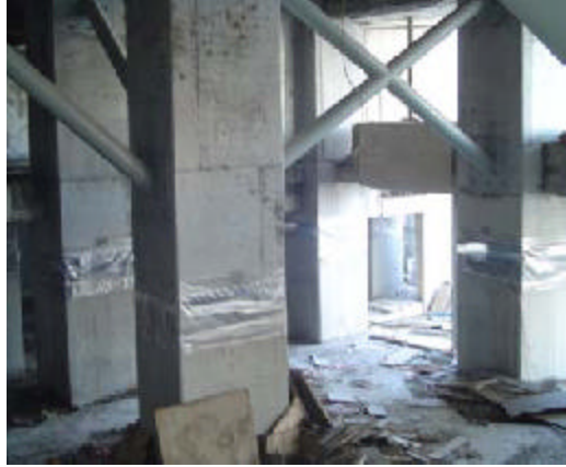
Figure 3.16: Diagonal bracings at the base level(Murat, 2006).
