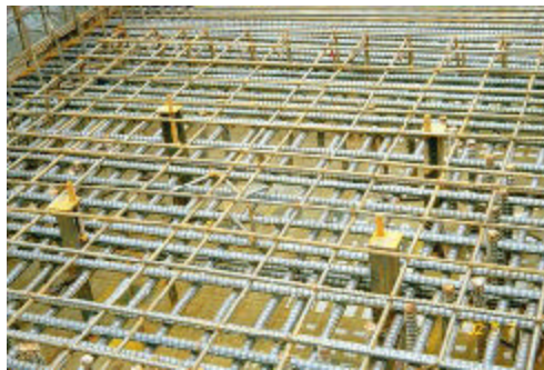
Figure 4.1: Installation stage (Dogan, 2007).
