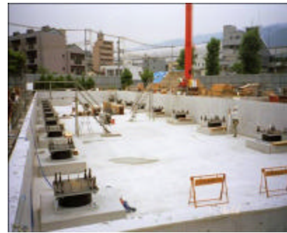
Figure 4.6: Mounted isolators (Em-Ke Ltd).
