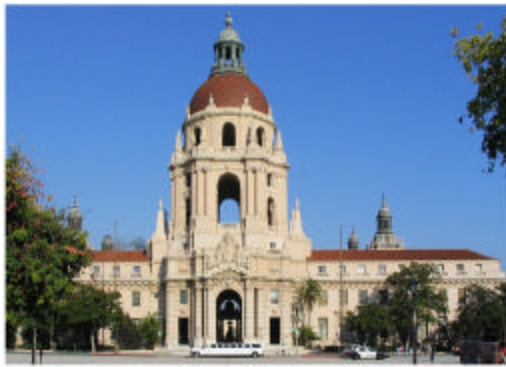
Figure 3.8: Pasadena City Hall (DIS, 2007).
