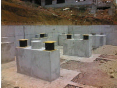
Figure 4.12: Isolators and pedestals, which connect dampers. Figure 4.13: Connection of damper to structure and pedestal (Lizundia, 2006).
