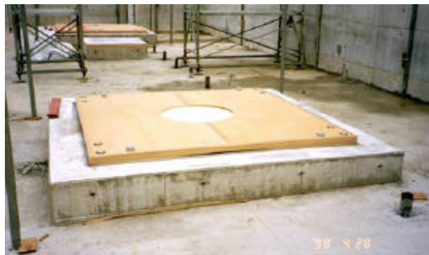
Figure 4.4: Grout pouring under the plate (Em-Ke Ltd).
