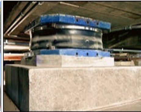
Figure 3.9: Isolation System for Pasadena City Hall (DIS, 2007).
