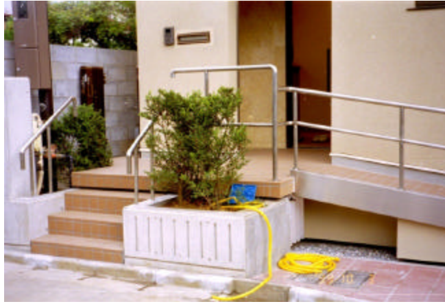
Figure 4.10: Staircase, which performing as cantilever in the base isolated building (Em-Ke Ltd).
