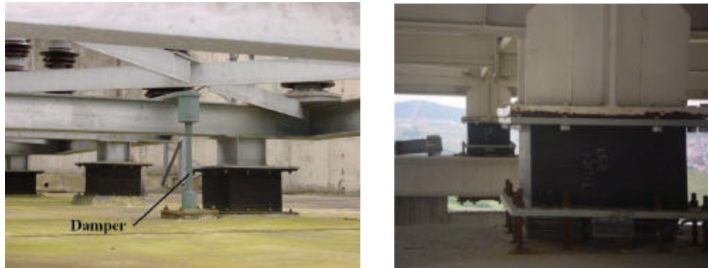
Figure 4.25: Steel beams for connecting isolators at base level (Robinson Seismic Ltd).
