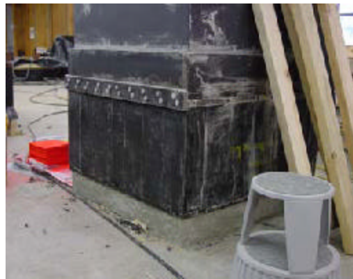
Figure 4.19: Installing isolator into its place (Robinson Seismic Ltd, 2003).
