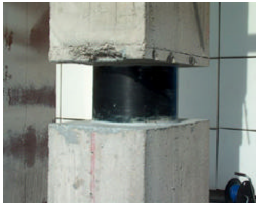
Figure 3.12: Installation of isolator in Antalya Airport (ERSE Company, 2009).
