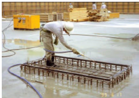
Figure 4.2: Concrete pouring of the foundation (EmKe Ltd).
