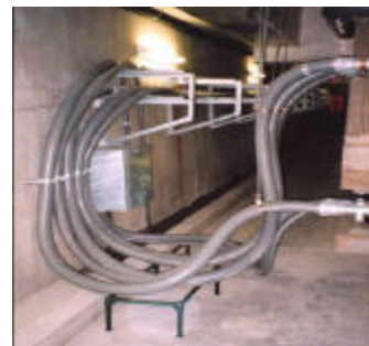
Figure 4.9: Isolating mechanical works in base isolated building (Em-Ke Ltd).
