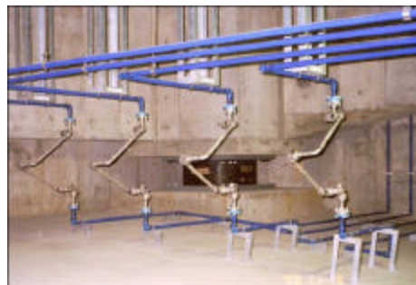
Figure 4.9: Isolating mechanical works in base isolated building (Em-Ke Ltd).
