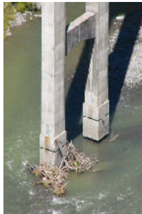
Figure 2.11: The pier base as built (Ma and Khan, 2008).
