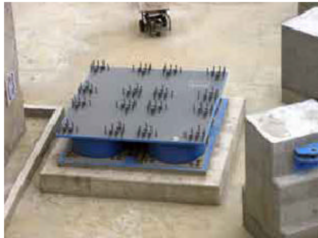
Figure 4.11: Group of isolators, which are located under a column with high vertical load (DIS, 2007).
