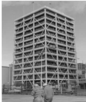
Figure 3.2: Union House, Auckland City (R.Park, 2000).
