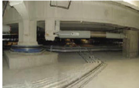
Figure 4.12: Isolators and pedestals, which connect dampers. Figure 4.13: Connection of damper to structure and pedestal (Lizundia, 2006).
