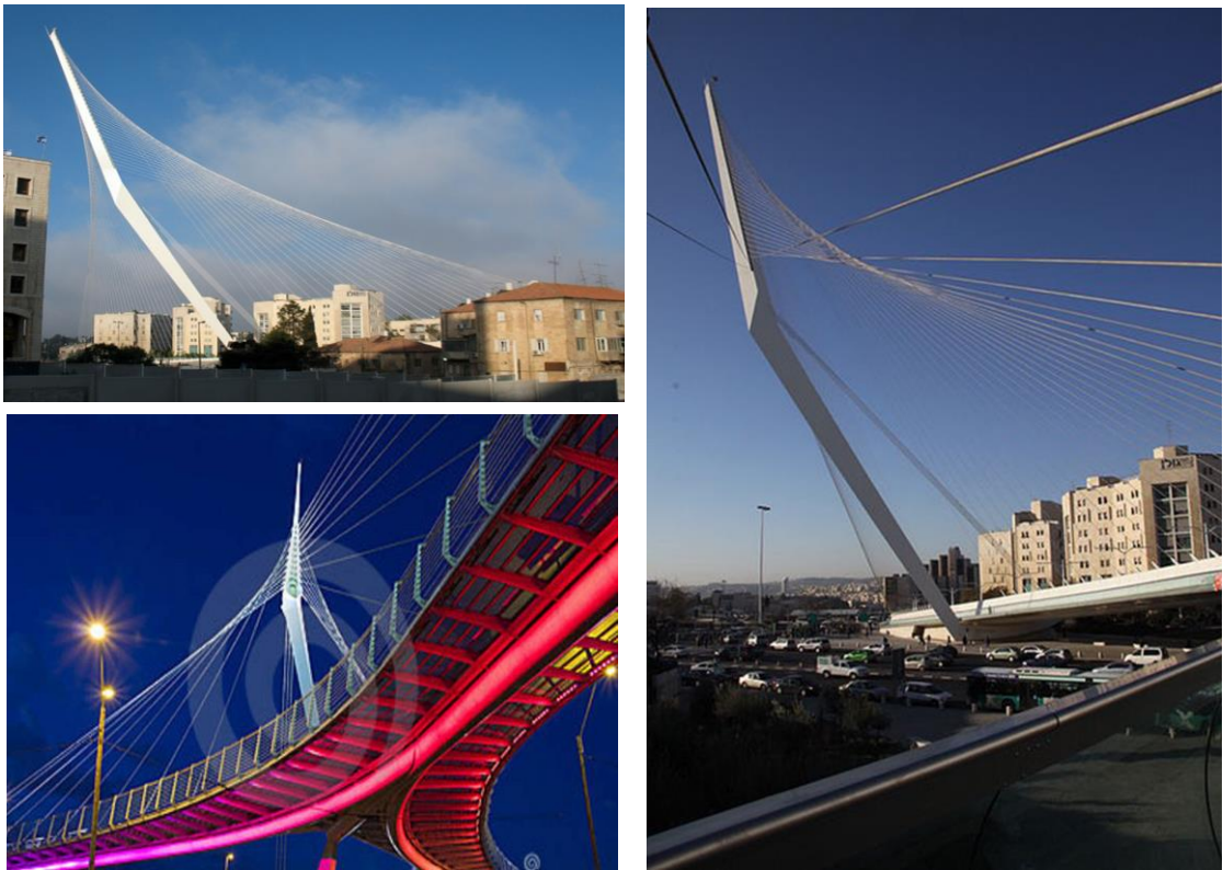
Figure 19: Jerusalem Chords Bridge in city of Petach-Tikva, Israel (Left Top: URL 26, Left Bottom: URL 27, Right: URL 7)
