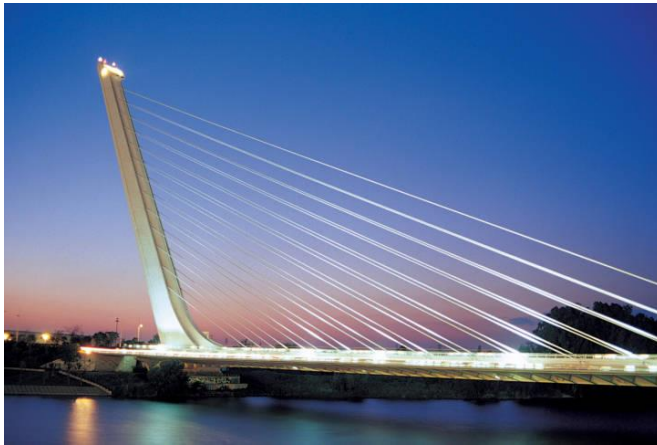
Figure 46: Alamillo Bridge in Seville, Andalusia, Spain, 1992 (URL 28)
