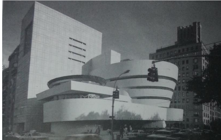
Figure 4.9: Solomon R. Guggenheim Museum and the extended block (Newhouse,1998)
