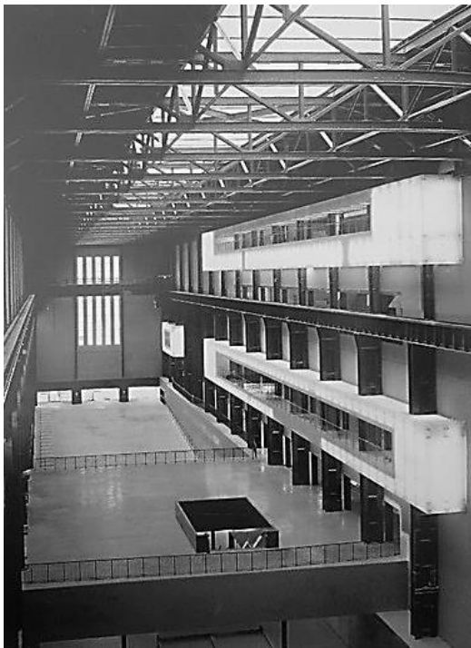
Figure 4.47: Ceiling opening in Turbine Hall, Tate Modern (Schittich, 2009)
