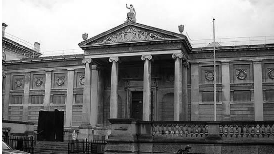
Figure 2.4: Ashmelean Museum Building, UK (McLachlan, 2006)
