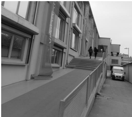
Figure 4.75: entrance ramp, Istanbul Modern Museum, Turkey (Author, 2012)
