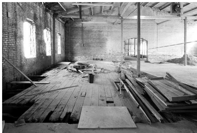
Figure 4.65: Building condition Before revitalization. Most of timbers are used in reused in new function (Architects and Artisans, 2011)
