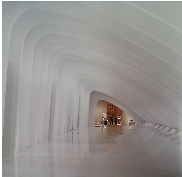
Figure 3.28: Linoleum flooring, Milwaukee Museum, USA (Tilden, 2004)
