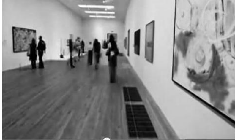
Figure 4.55: floor ventilation system, Tate Modern (Olins, 2010)
