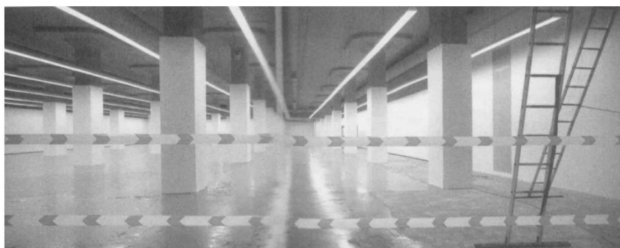
Figure 4.73: Istanbul Modern during the restoration (Istanbul Modern Library catalogue, accessed in 2012)
