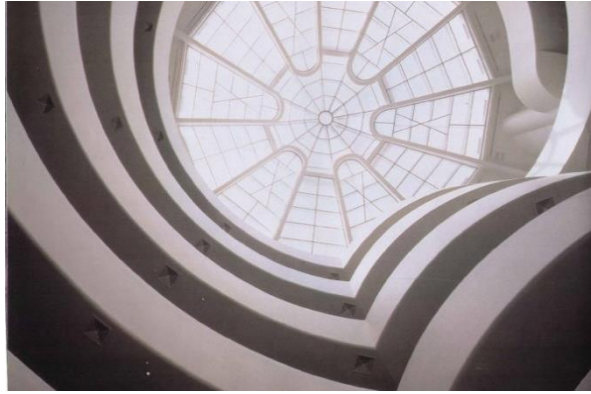
Figure 4.21: Matt glass and air conditioning system, Solomon R. Guggenheim Museum (Tilden,2004)
