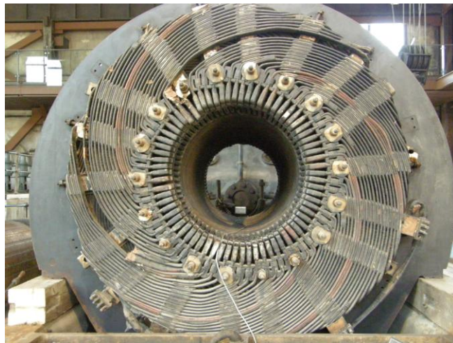
Figure 2.16: Santralistanbul Museum's Machinery System after Conservation, (Türker, 2008)
