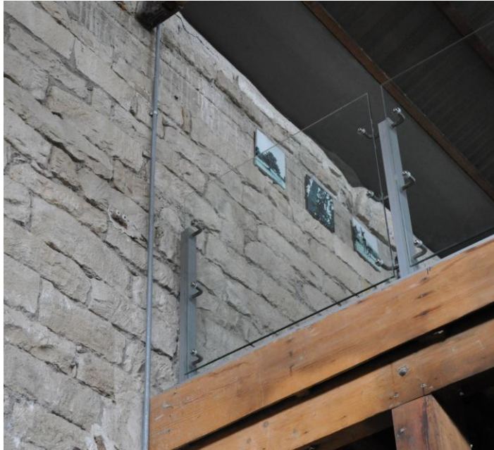
Figure 2.31: Mezzanine of the Museum (Türker archive, 2010). Transparent Balustrade has been used to Avoid Disturbing the Unity of the Building.
