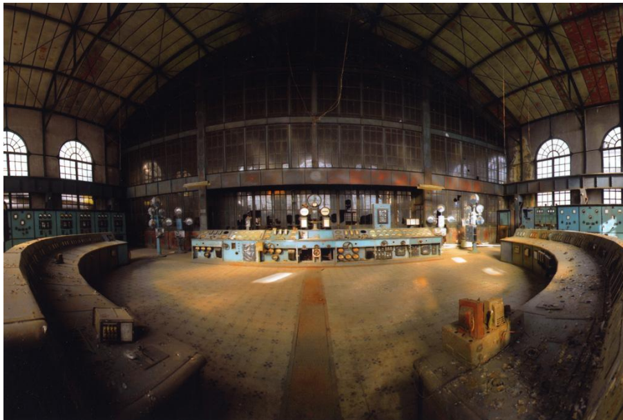
Figure 2.13: Control Room of Silahtarağa Power Station (Bilgi University Archive, 2010)
