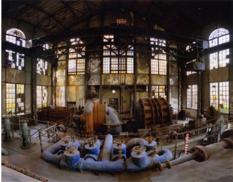
Figure 2.12: Silahtarağa Power Station Interior Space before Conservation (Bilgi University Archive, 1986)
