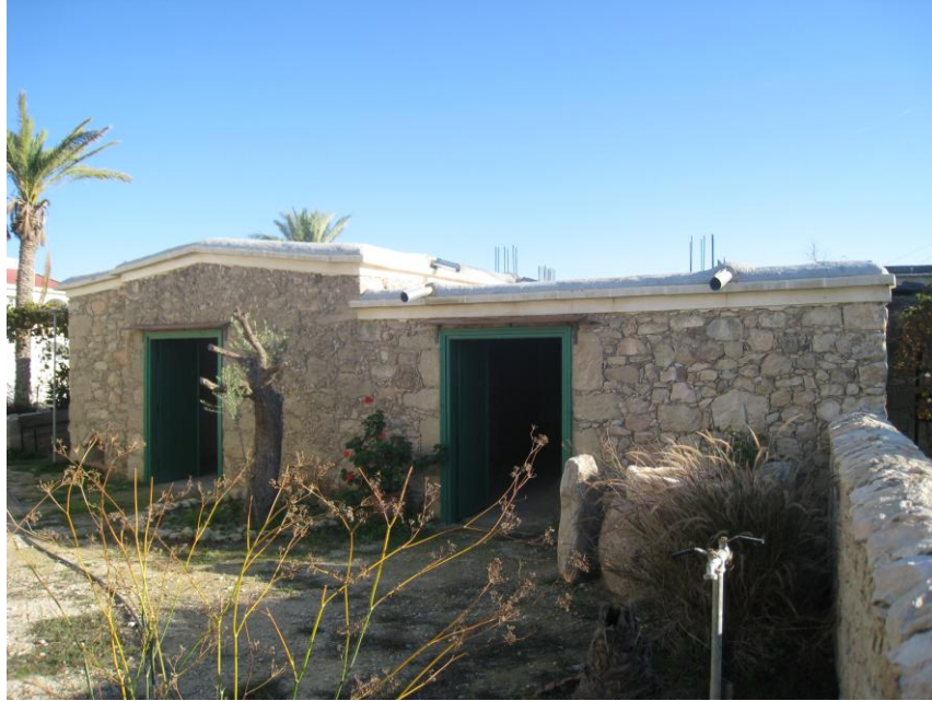
Figure 3.10: Büyükkonuk Olive Oil Mill Building after Conservation (Golmakani archive, 2009)
