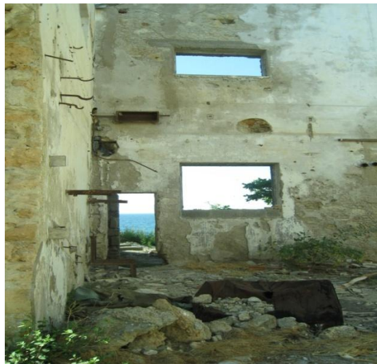
Figure 4.19: Former Machines Room of Zeyko Olive Oil Factory, Kyrenia (Golmakani archive, 2009)
