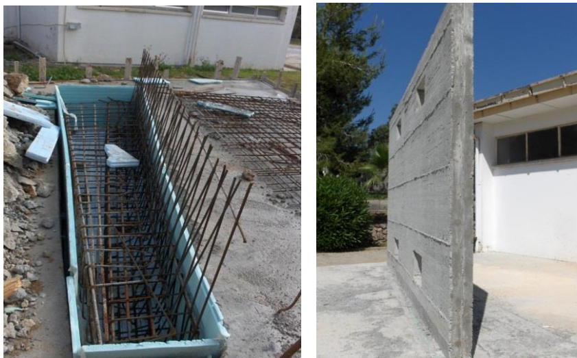
Figure 6.5. Foundation construction procedure of TSW
