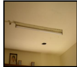
Figure 3.54: ceiling is reinforce concrete in Halil Kara Coffeehouse. (By author)
