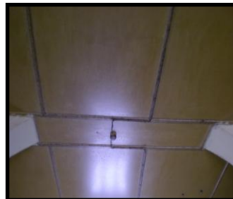
Figure 3.53: plywood board ceiling in Erdogan İktas Coffeehouse. (By author)
