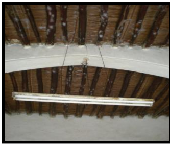
Figure 3.52: wooden beams and dry-reed material in Yusuf Soykara Coffeehouse. (By author)
