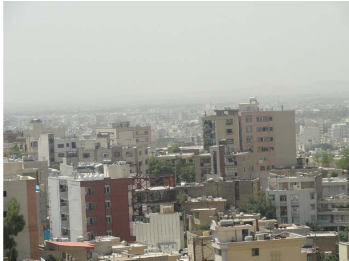
Figure 3.14.Lack of Porosity in Shiraz Urban Space
