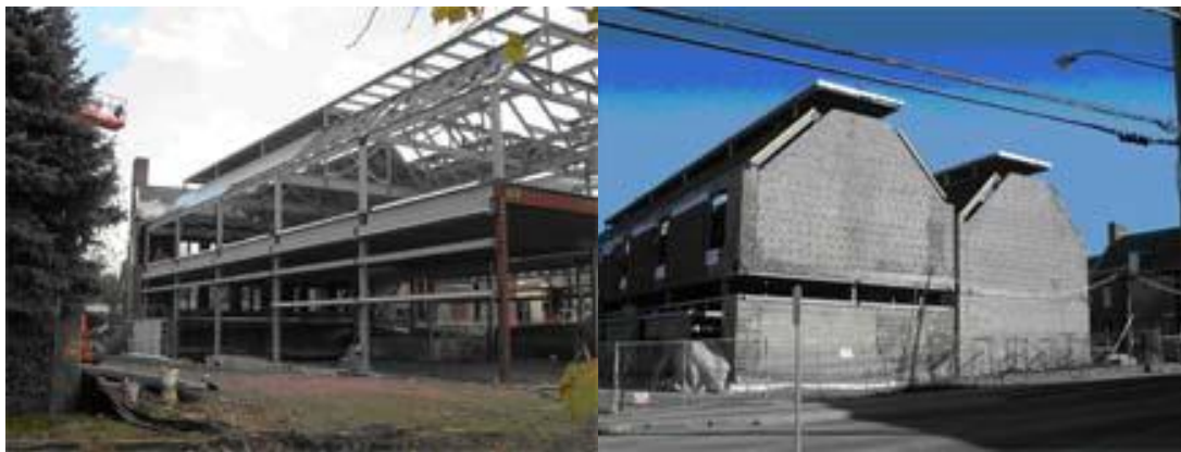
Figure 3.2: Structure of Hamilton Avenue School
