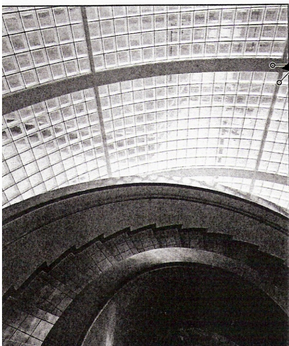
Figure 9.8 Staircase enclosure built with glass masonry units.
