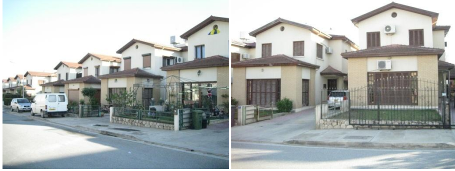
Figure 35: Levent houses in Ortaköy district (Author, 2011)
