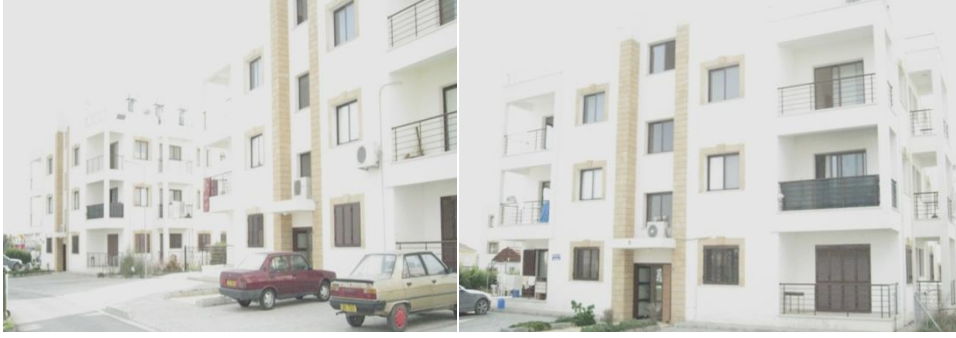
Figure 38: Levent Apartments in Gönyeli district (Author, 2011)
