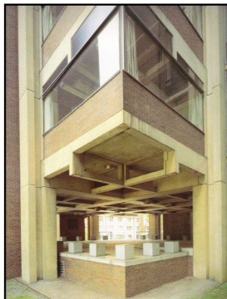
Figure 4.16: ground floor entrance showing Vierendeel trusses empty of servant services such as mechanical ducts (Brownlee & De Long, 1991, p.177)
