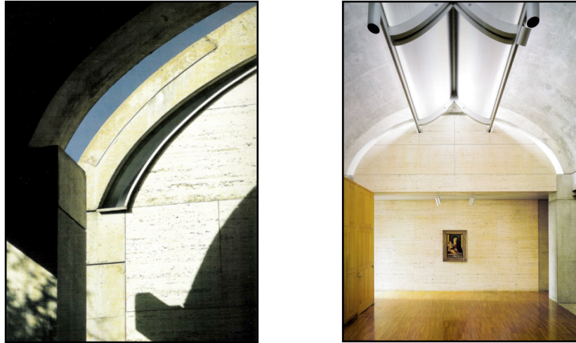
Figure 4.52: Exterior and interior of cycloid vaults, showing using glass between wall and vault to indicate the non-load bearing cycloid vaults. (McCarter, 2005, p.350)
