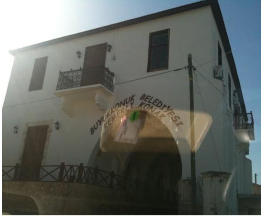
Figure: 33. Village – Style Accommodation
