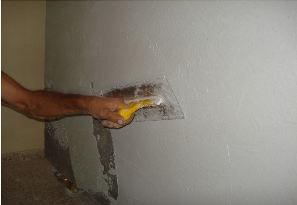
Photo 3.38: Third Coat Plastering (Ready-Mixed) (Final Coat) Applied on Wall Specimen.
