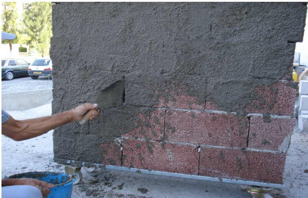
Photo 3.35: First Coat Plastering Applied on Wall Specimen.
