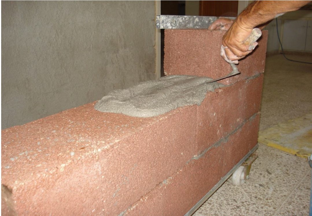
Photo 3.32: Construction of Wall Specimens.
