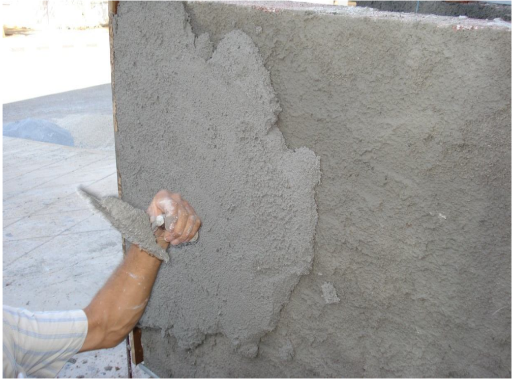
Photo 3.36: Second Coat Plastering is Applied on Wall Specimen.
