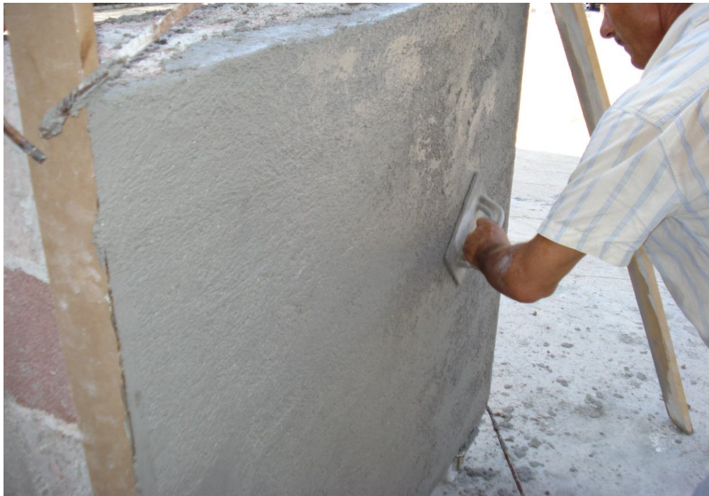
Photo 3.37: Finishing of Second Coat Plastering.
