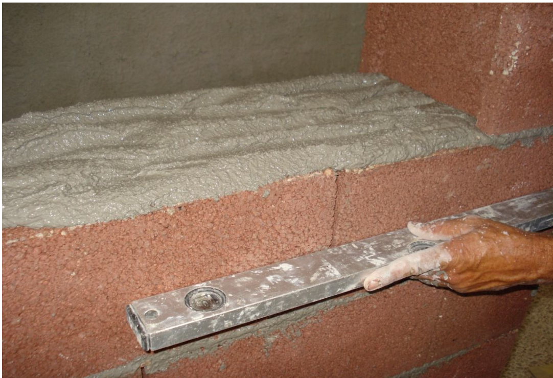
Photo 3.33: Levelling of Walls.
