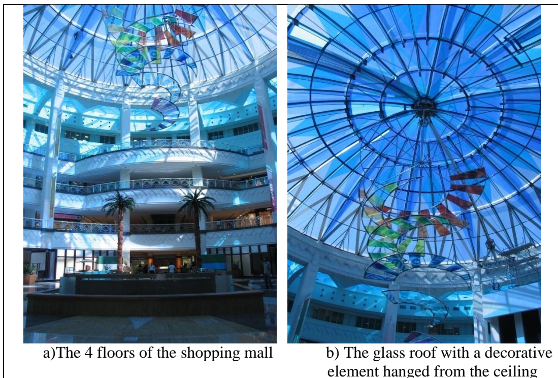
Figure 36: The glass roof of Oasis Center Mall
