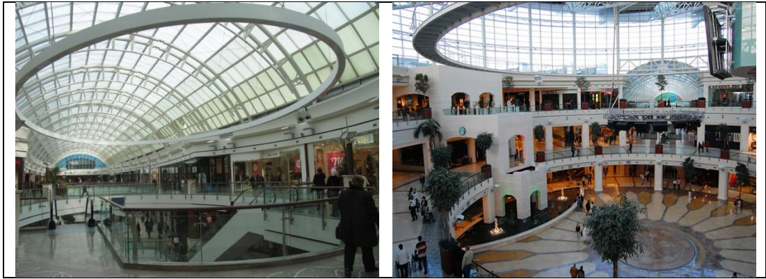
Figure 66: The glass roof of Istinye Park Mall
