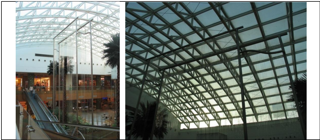
Figure 41: The glass roof of Times Square Center Mall
