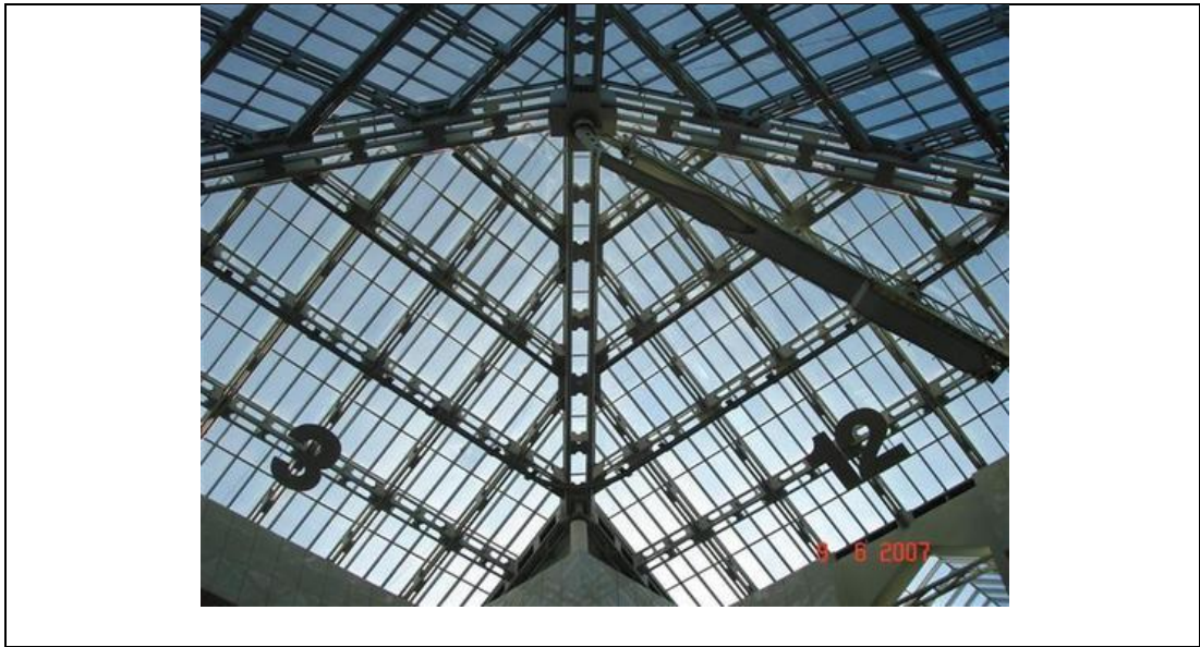
Figure 80: The glass roof of Cevahir Mall
