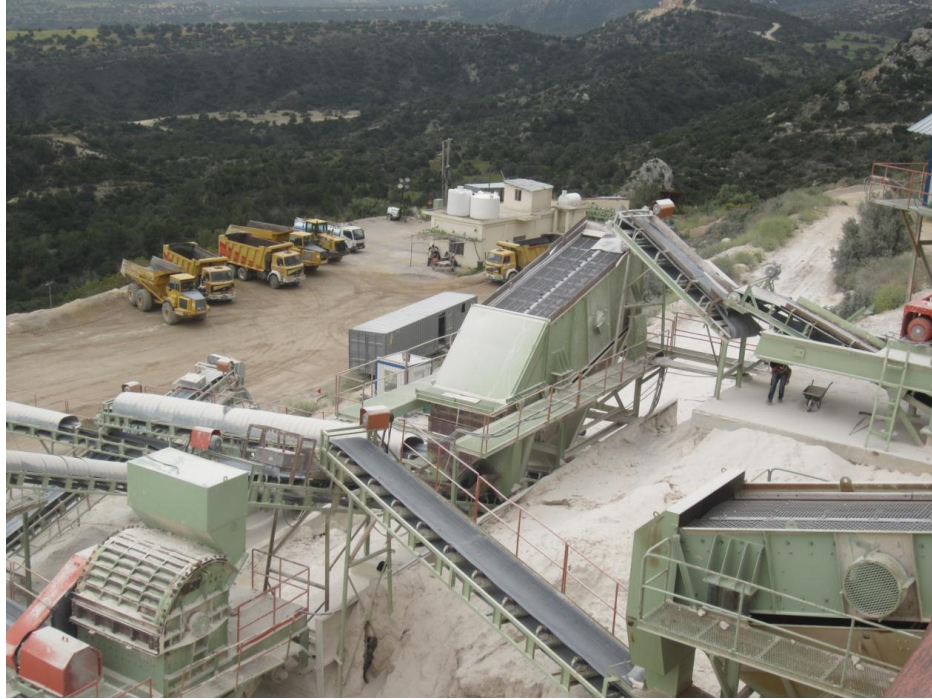
Figure 2: Overlooking of jaw crusher
