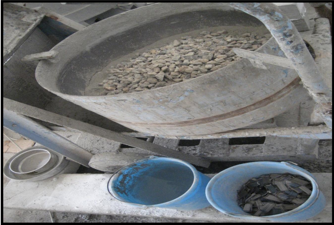
Photo 1: The mixer and the materials ready for mixing
